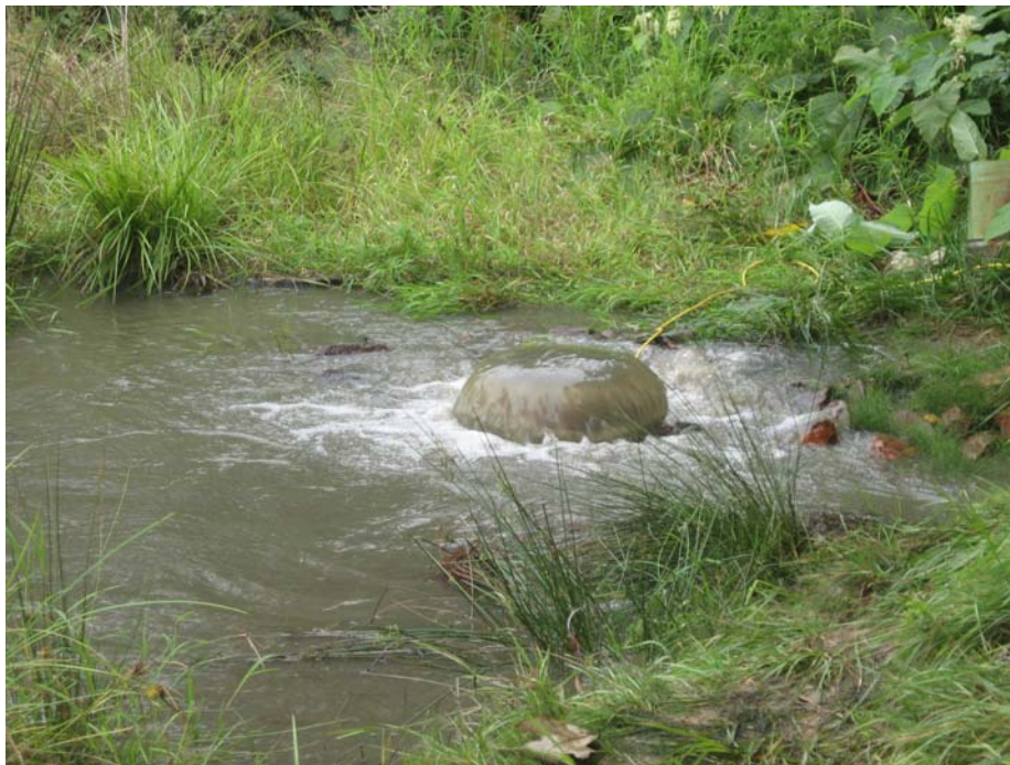
Photo 3. The large flow of water immediately after removal of the borehole obstruction.
