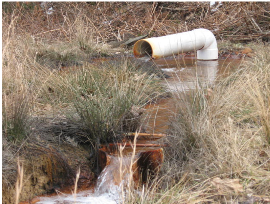
Photo 1. Wolford Run borehole discharge and flume.
