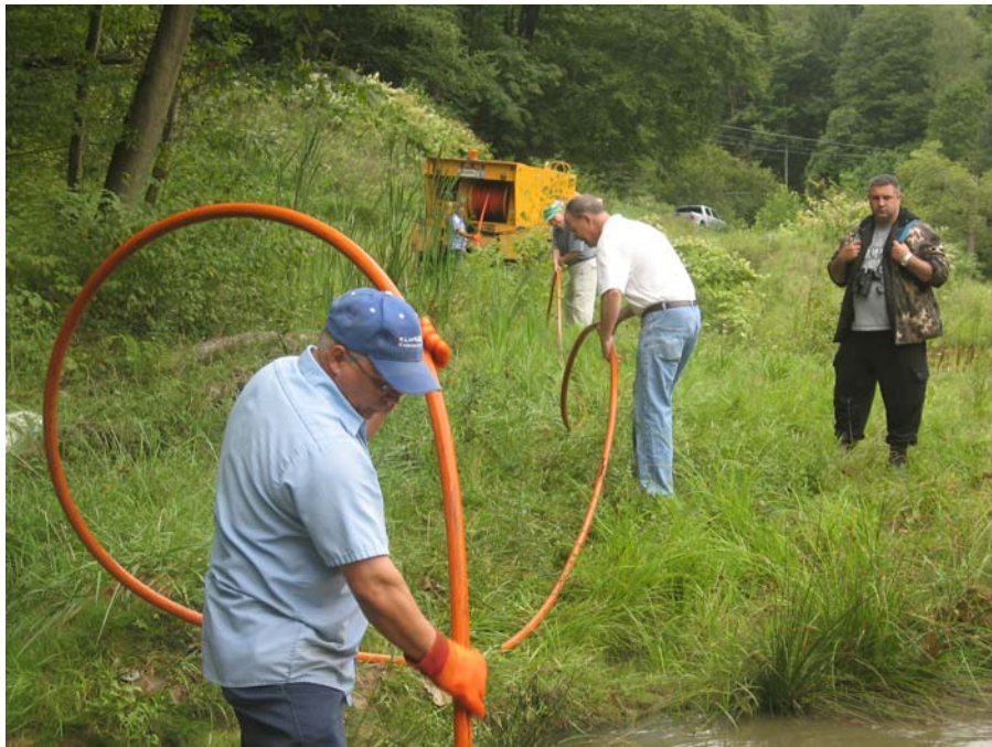
Photo 2. Kiski Water Authority crew feeding plastic tubing into the borehole for purpose of removing blockage.
