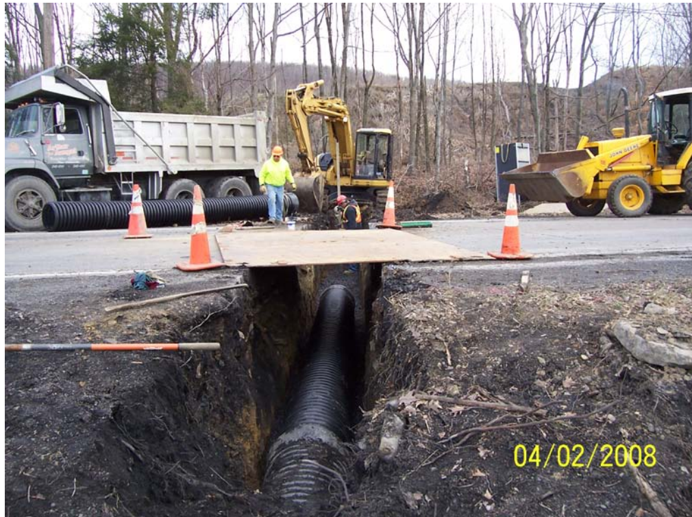
Picture 15. Placement of primary settling basin intake pipe under highway.
