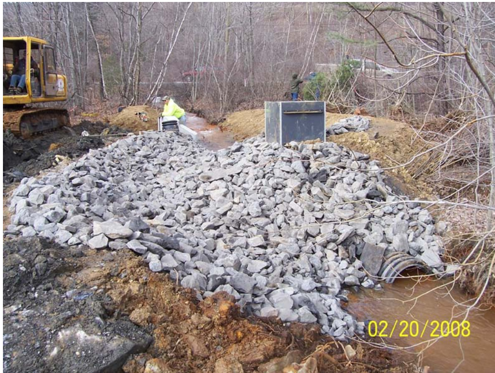
Picture 5. Placement of water level control structure in discharge channel.
