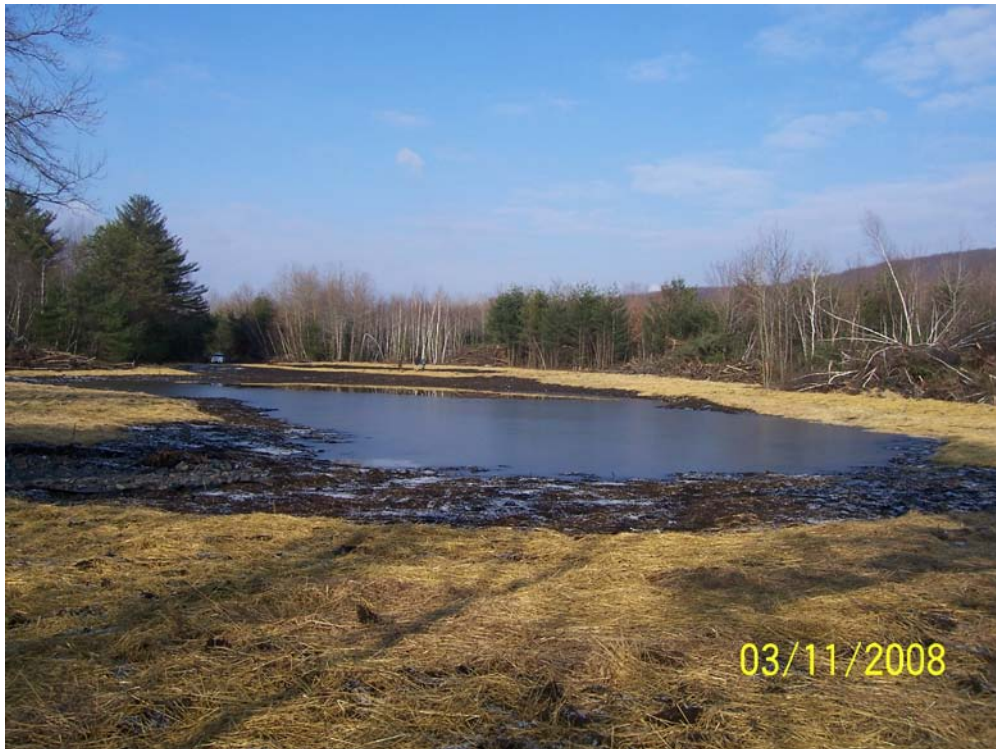
Picture 11. Completed polishing wetland, before being filled with water
