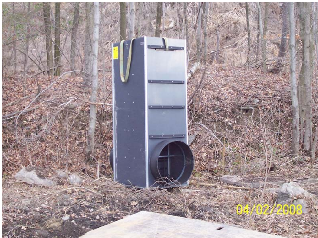
Picture 4. Inline water control level control structure to be placed in discharge channel.
