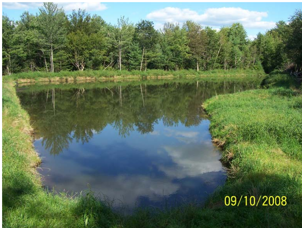
Picture 8. Overflow settling basin receiving water from the primary settling basin.
