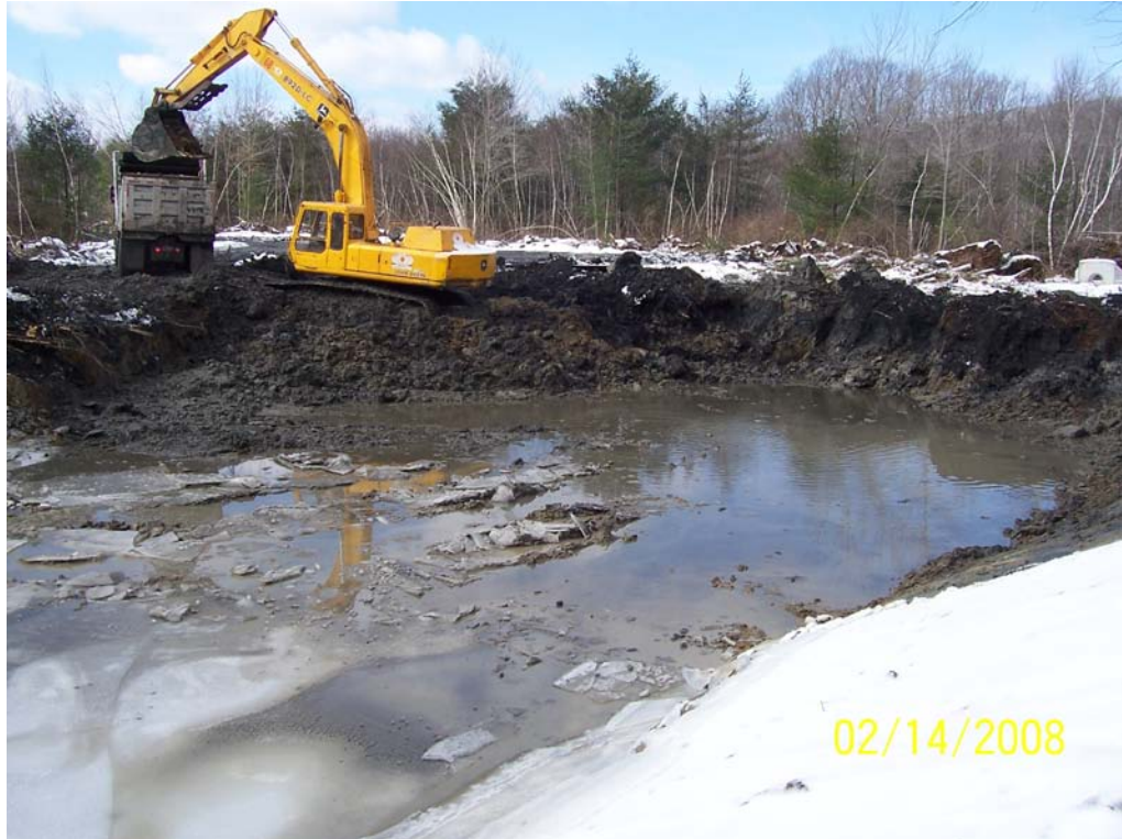
Picture 2. Excavation of the overflow settling basin
