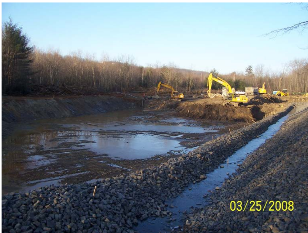
Picture 14. Excavation of the primary settling basin.
