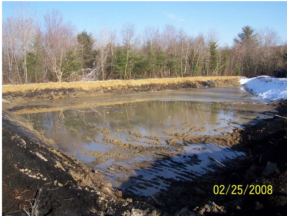
Picture 7. Completed overflow settling basin before being filled with water.
