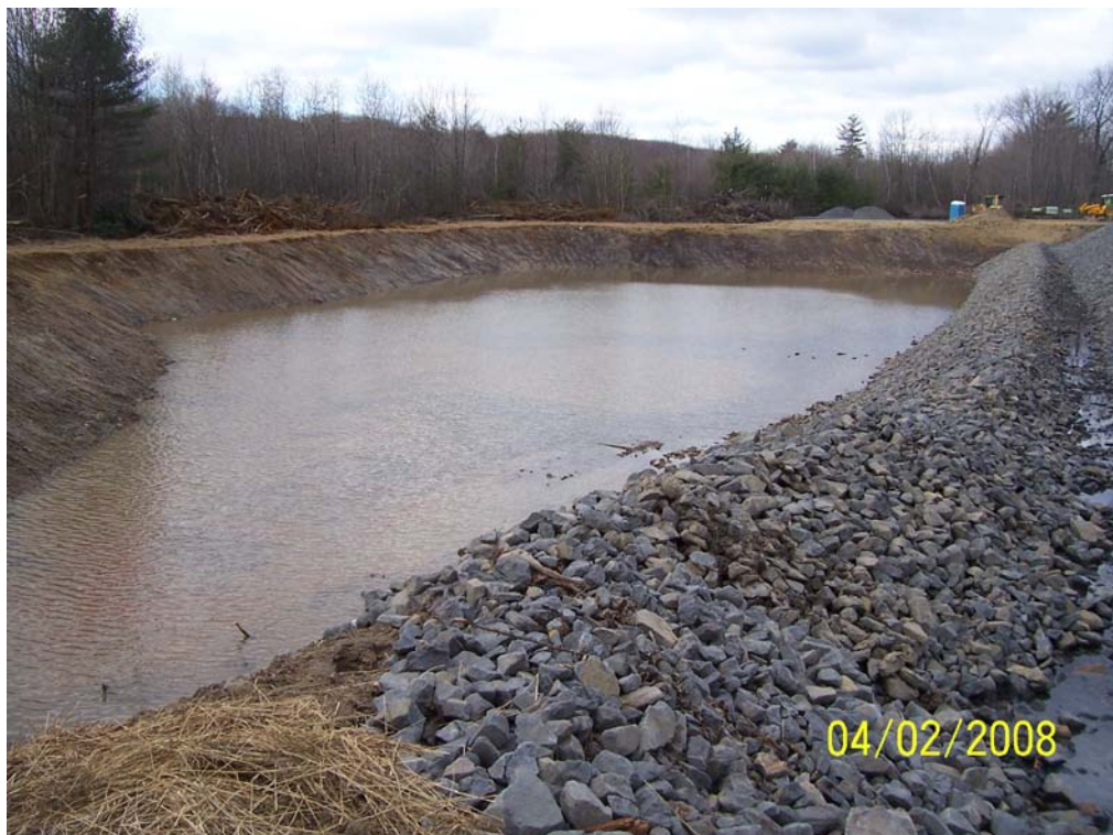
Picture 16. Completed primary settling basin before being filled with water.
