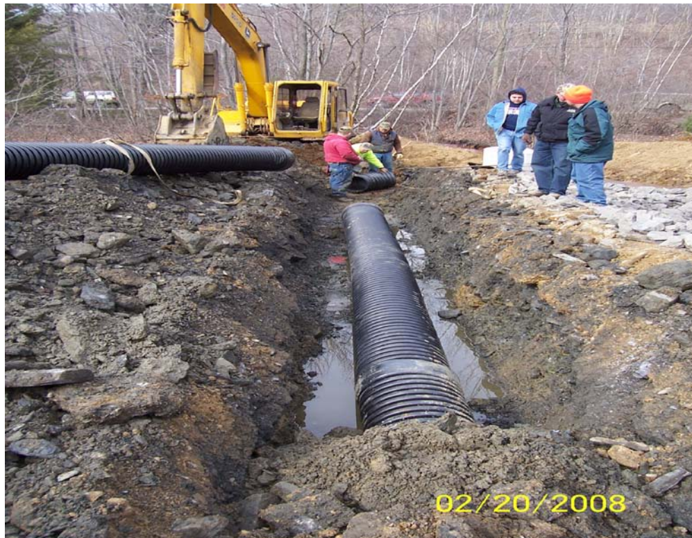
Picture 6. Placement of overflow settling basin intake pipe.
