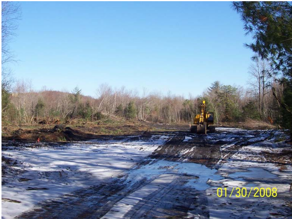
Picture 9. Clearing and grubbing of the polishing wetland site.
