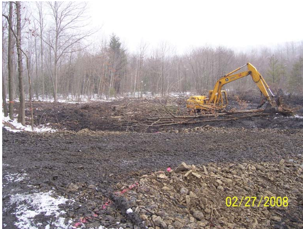
Picture 13. Clearing and grubbing of the primary settling basin site.
