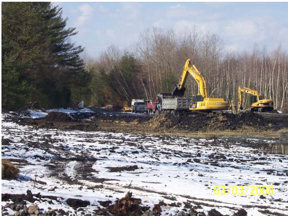
Picture 10. Excavation of the polishing wetland.
