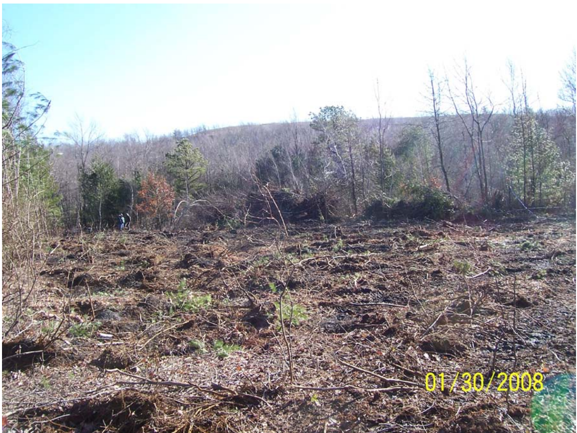
Picture1. Clearing and grubbing of the overflow settling basin site.
