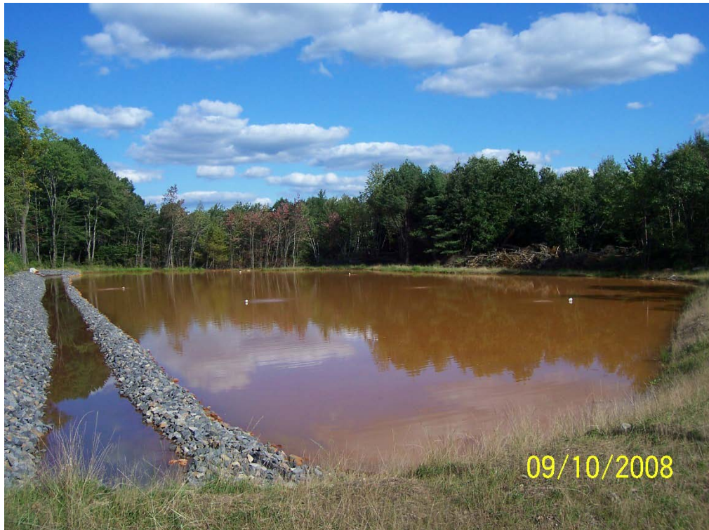
Picture 17. Primary settling basin receiving discharge water and operating aeration system.
