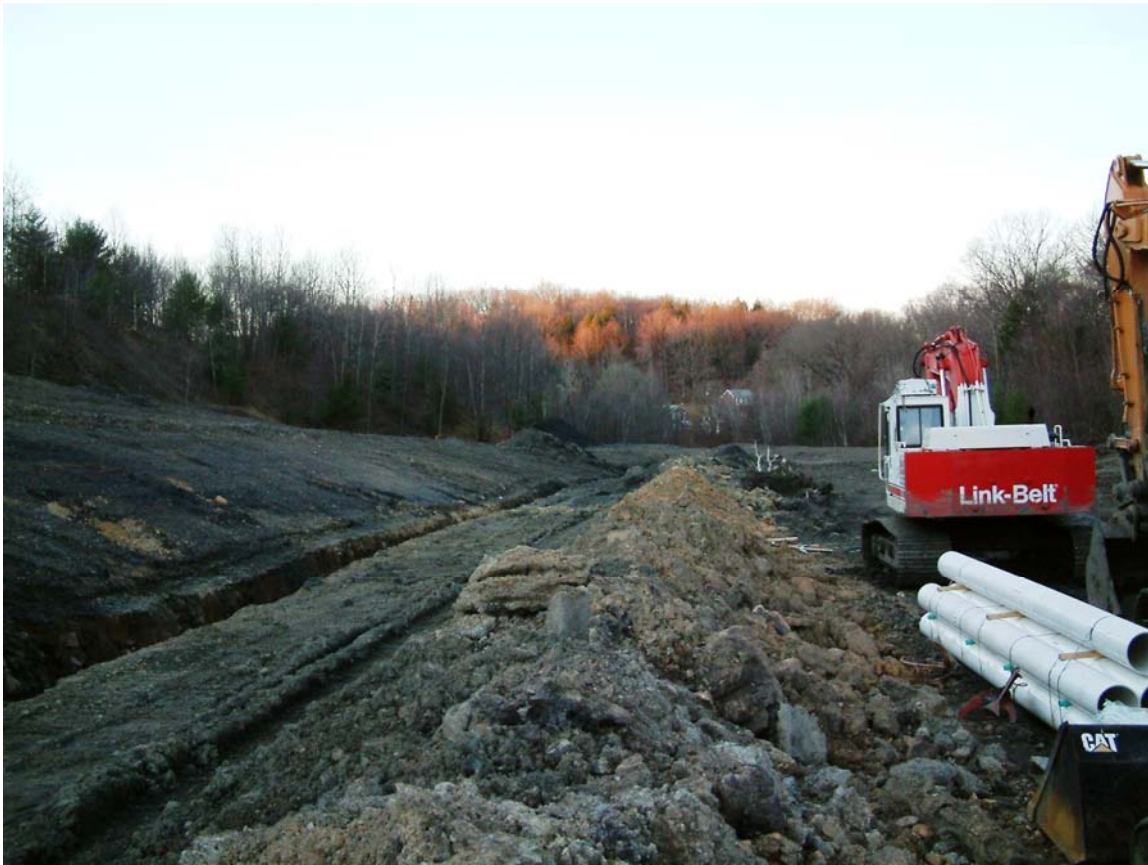
Photo 5: Start of construction of anoxic limestone drain (ALD).
