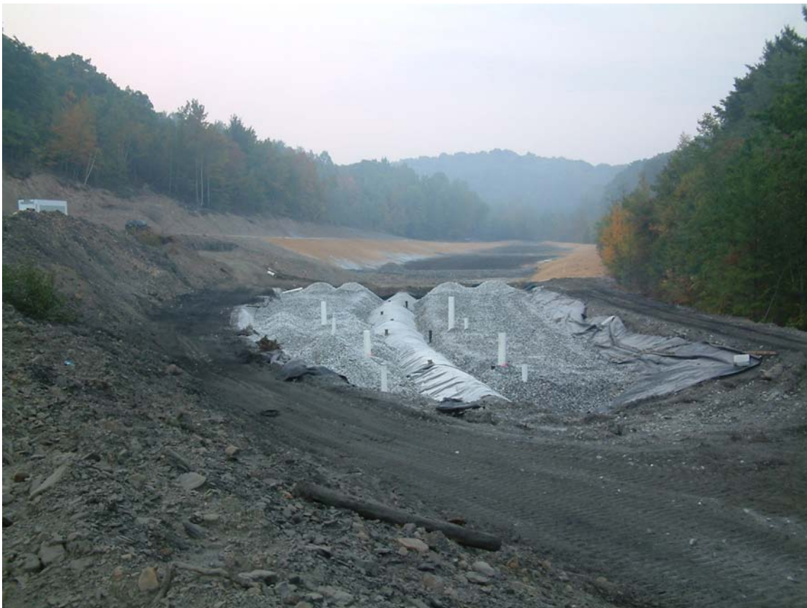
Photo 14: Completed ALD prior to covering with HDPE 40 mil liner and topsoil.
