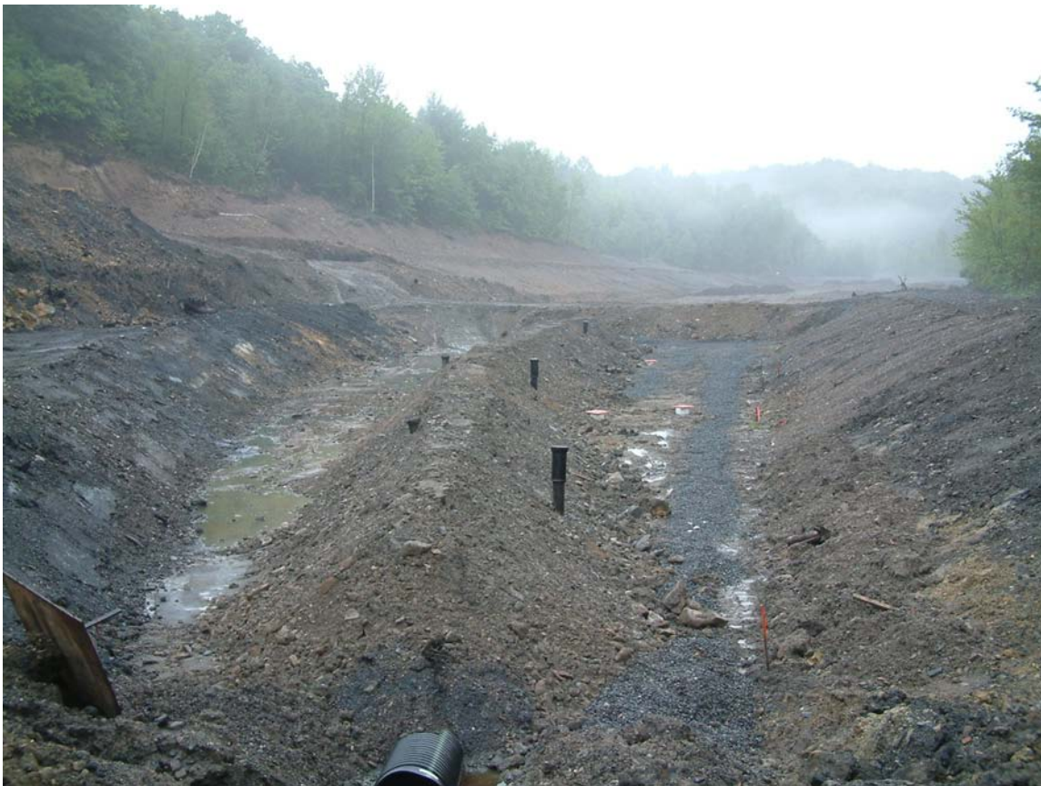
Photo 8: Beginning of installation of piping for ALD.
