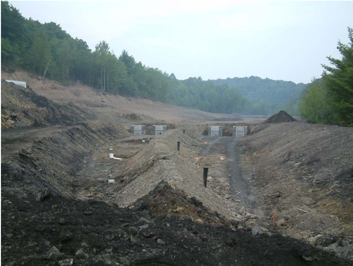
Photo 9: Installation of concrete outflow control structures in ALD.
