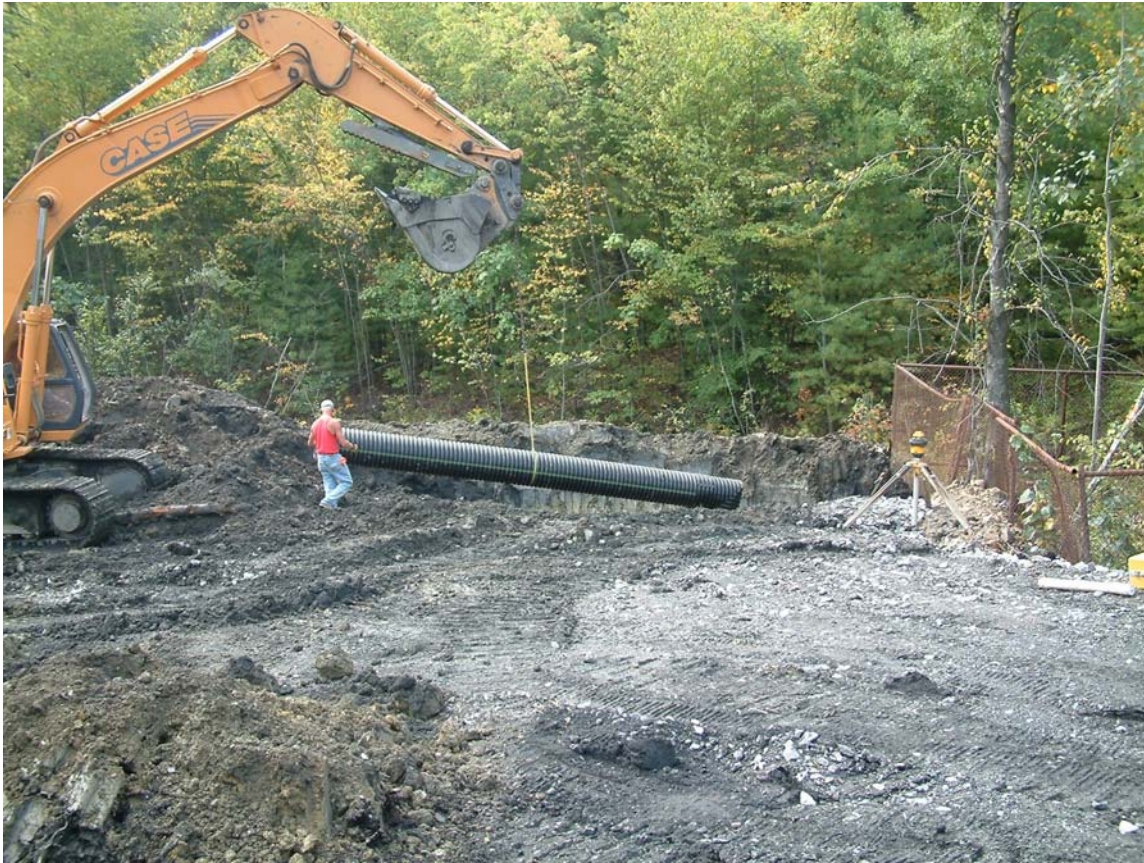
Photo 13: Installation of inflow pipe from discharge to ALD.
