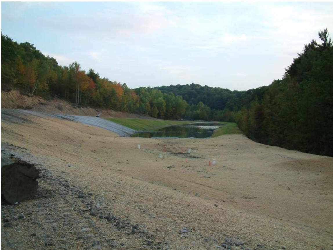
Photo 16: Completed treatment system during final seeding and mulching. View is looking south with ALD in foreground.
