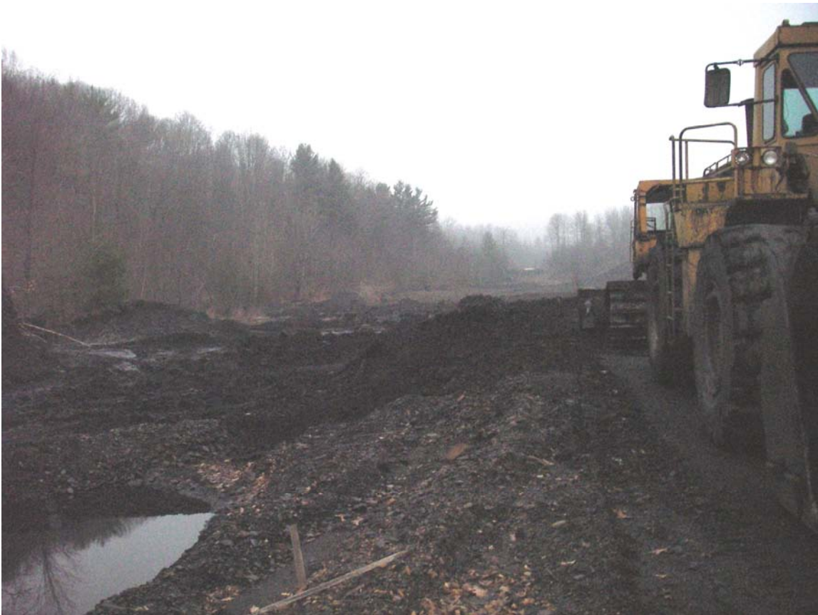
Photo 2: Clearing & grubbing of project site prior to construction.
