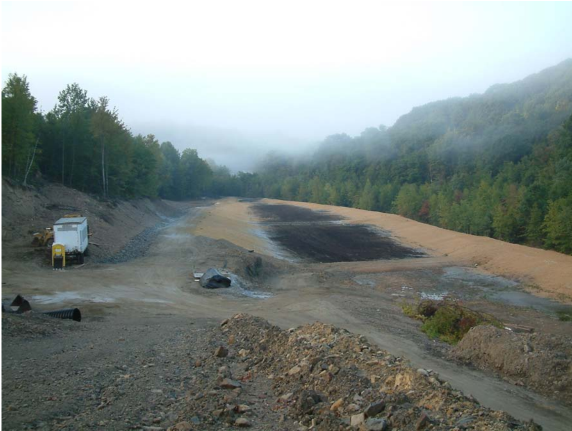
Photo 11: Completed wetland treatment cells following seeding and mulching.
