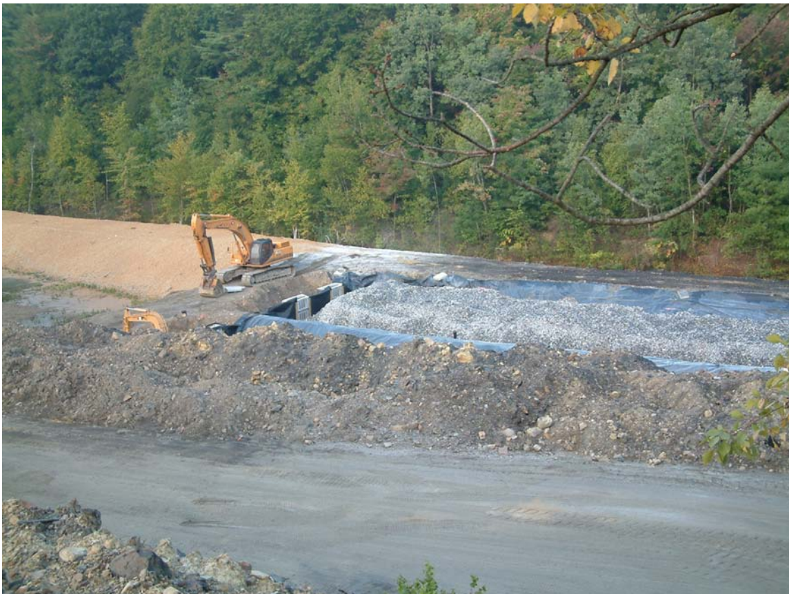
Photo 12: Installation of limestone in the ALD.
