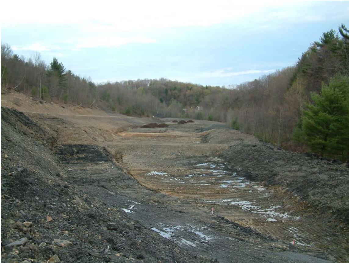
Photo 7: View of construction of ALD with wetland cells in background.
