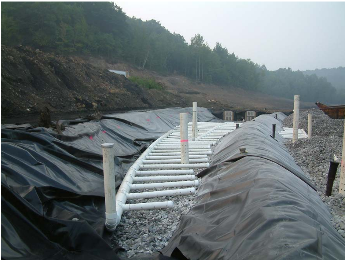
Photo 10: Completion of pipe installation and limestone addition to ALD.
