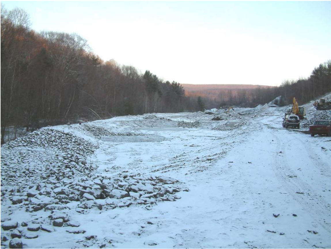
Photo 3: Rough grading of project site for construction of treatment system cells.
