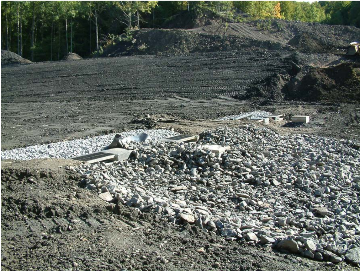
Photo 15: Completed ALD outflow structures.
