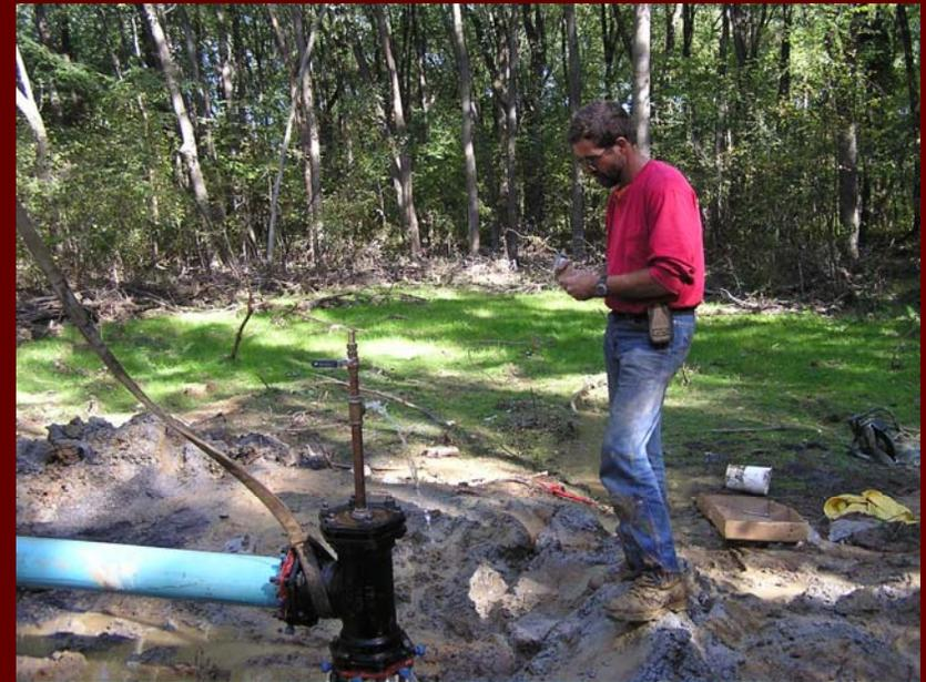
The pilot borehole was capped and encased in a concrete vault. That vault will protect from vandalism and weather. It also enables easy access for sampling.
