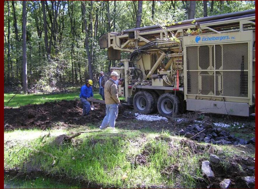
**Part II – Hole #1 being drilled by Eichelberger Drilling on October 6<sup>th</sup>. The drill rig moved 175 feet down without encountering a mine void or artesian flow.**
