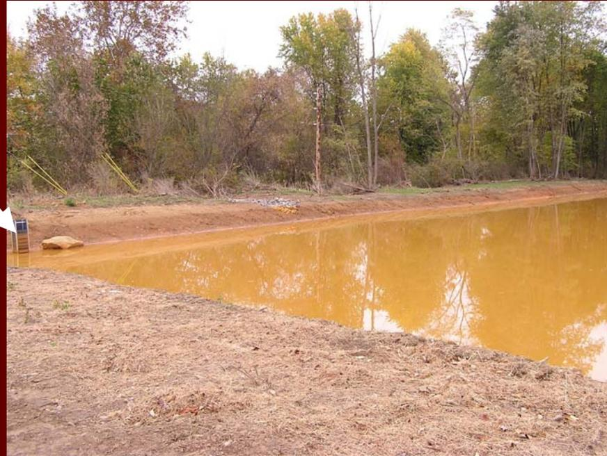
The pond shown after collecting water from the drilling process. The purpose of the pond was to gather water and allow iron oxide the opportunity to settle prior to water entering the Loyalhanna Creek.
