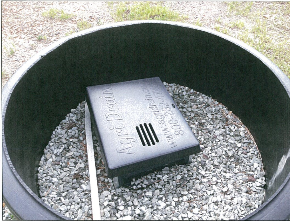
Photo 7: Inline Water Level Control Structure in Casing
