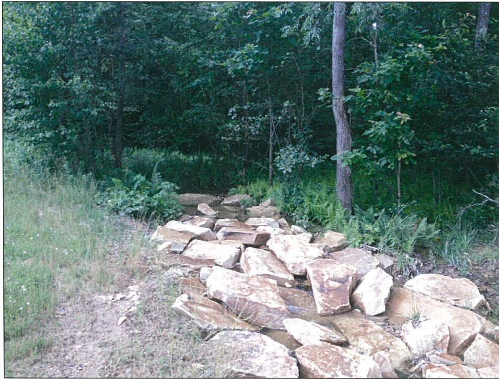
Photo 6: Rock Channel Lining at Channel 3
