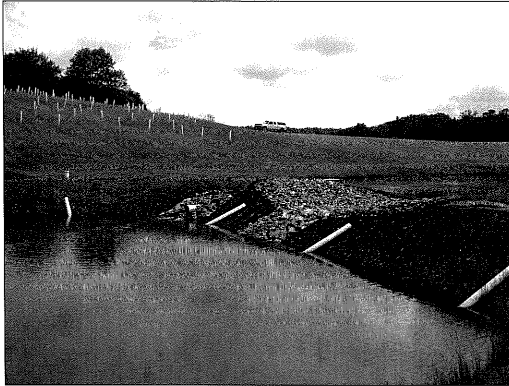
Photo 4: Vertical Flow Pond/Limestone Cell 2 (VFP2) with Underdrain Cleanout Ports
