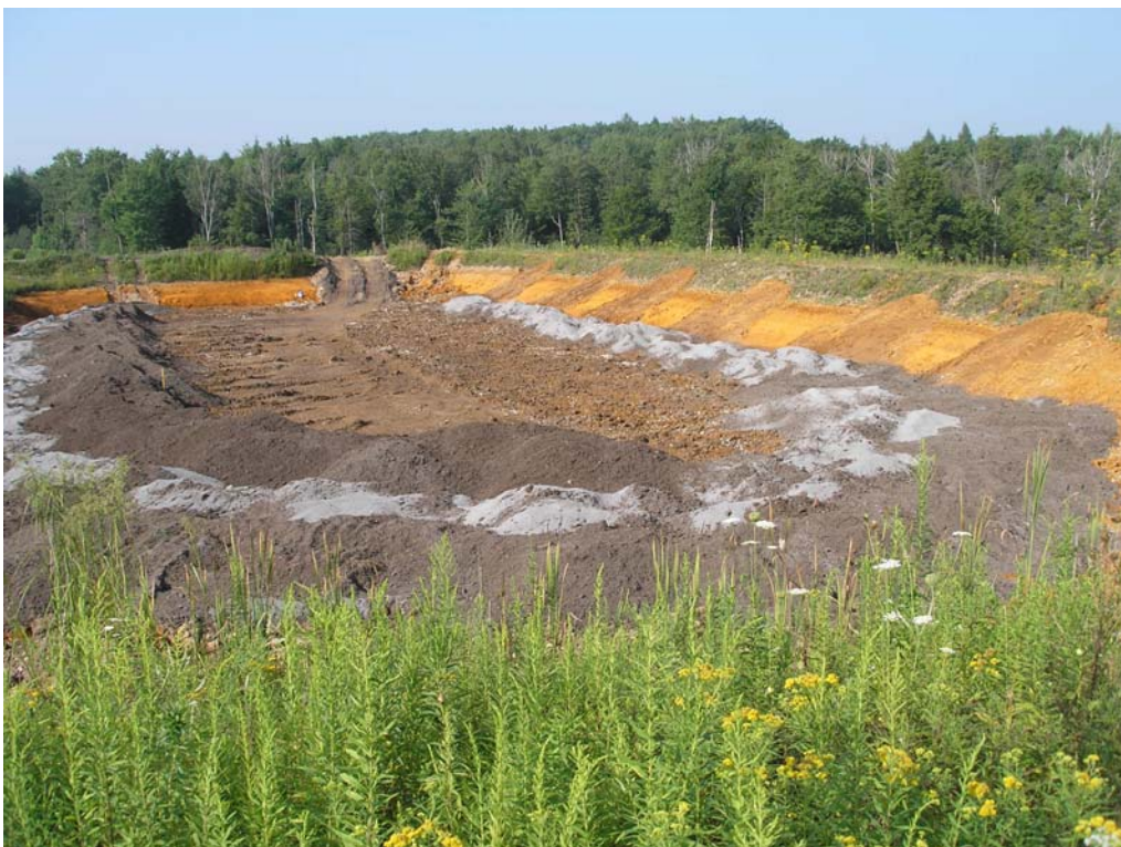
Photo 2. VFP 1 after removal of Fe precipitate and partial addition of new compost.
