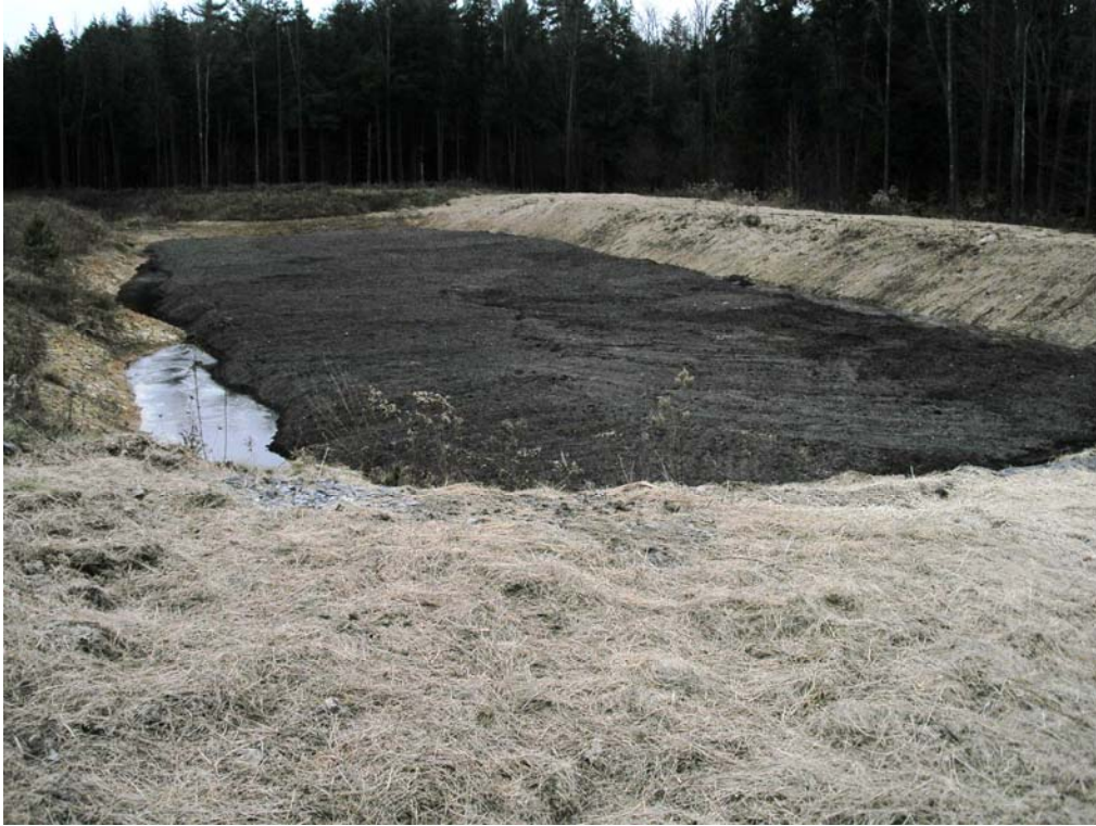
Photo 7. VFP2 after completion of compost addition.
