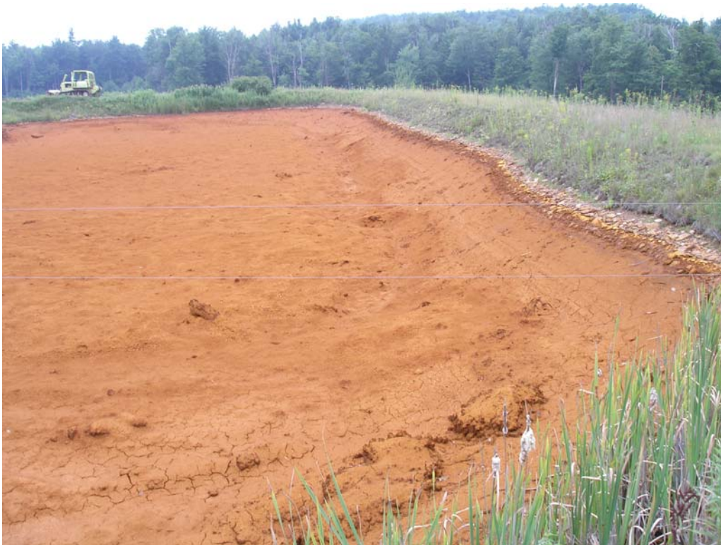
Photo 1. VFP 1 after draining, showing Fe precipitate.
