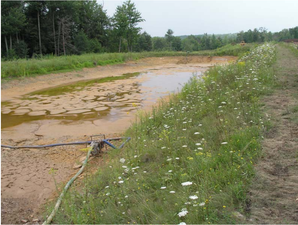
Photo 5. VFP 2 after draining, showing Fe precipitate.
