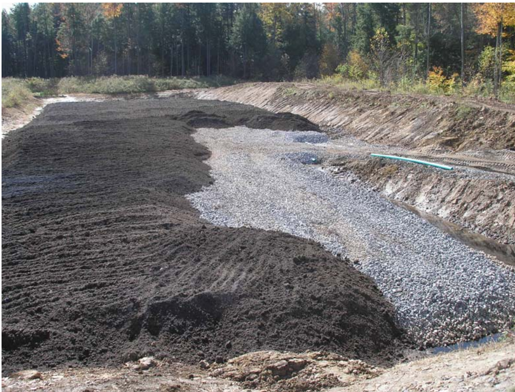
Photo 6. VFP 2 after emplacement of new limestone, underdrain and part of compost.
