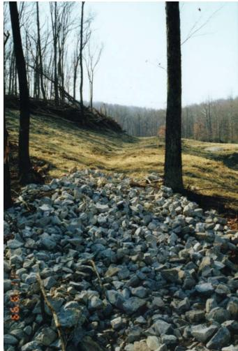
Above: Diversion ditch (looking northerly) preventing surface water runoff from entering the passive treatment system. (11/19/99)
