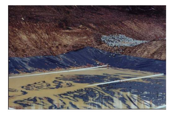
Underdrain of Vertical Flow Pond before addition of limestone and compost. (11/3/99)
