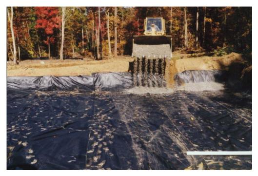
Sandstone aggregate being placed to bed pipe for outlet manifold in Anoxic Limestone Drain. (10/1999)
