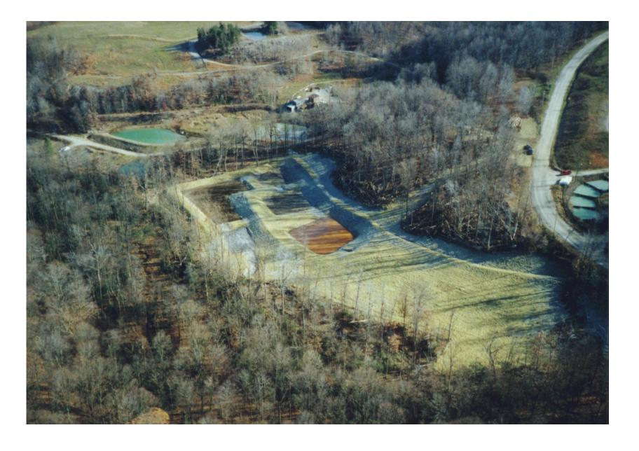
Aerial view of passive treatment system for Phase I constructed in 5 weeks 10/11/99 through 11/17/99 taken one day after construction. (Photo take 11/18/99 by Ron Horansky, MCI, PA DEP, Greensburg, DMO)
