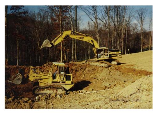
Construction of 500 ton Horizontal Flow Limestone Bed. (11/9/99)
