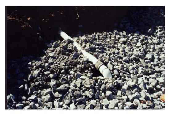
Influent pipe from Anoxic Collection System to Anoxic Limestone Drain. (10/28/99)
