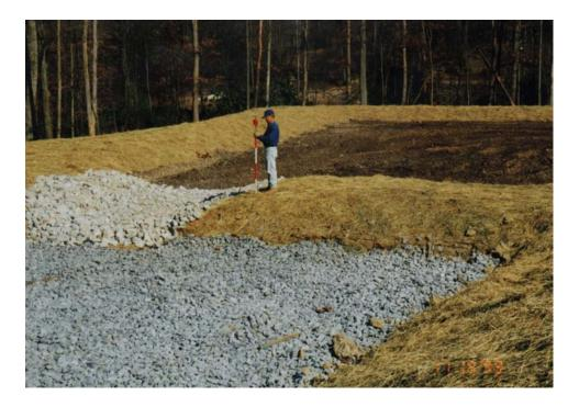
Spillway from 11,000 SF Wetland to Horizontal Flow Limestone Bed containing 500 ton of AASHTO #1 aggregate. Rodman surveying for "As-Builts." (11/19/99)
