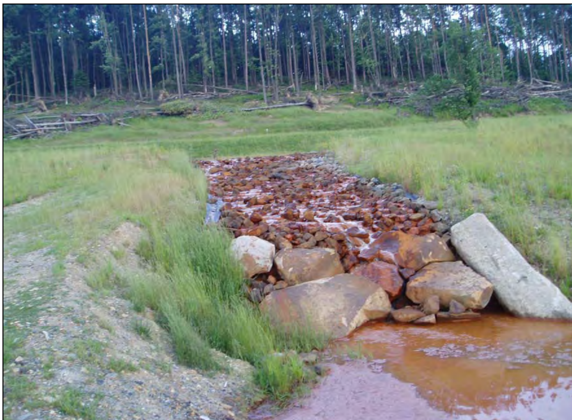
Settling Pond 3 ( Above ) receives influent from Wetland 1. A baffle curtain was installed to decrease short-circuiting and to increase retention time before discharging into Wetland 2 via a rock-lined spillway ( Below ).
