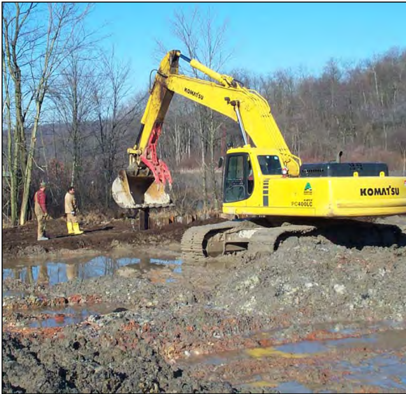
John Stoops, Mike Colosimo, and Kevin Stiner of Quality Aggregates installing Z-piling in order to maintain pre-project stream elevation from existing beaver dam across Seaton Creek at the “narrows” between the Flick and L-shaped gob piles. (3/28/02)
