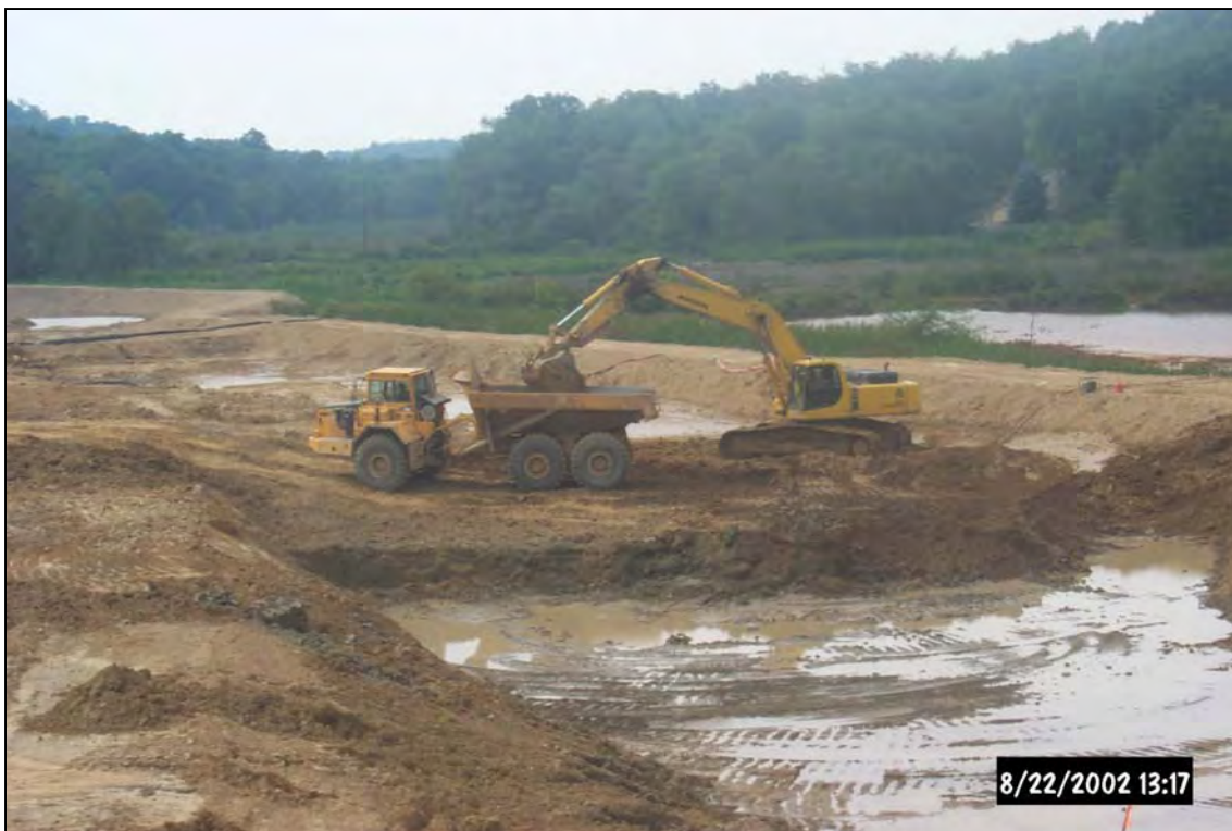
Excavation for Horizontal Flow Limestone Bed required substantial “dirt moving”.
