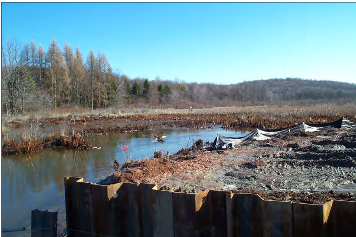
John Stoops, Mike Colosimo, and Kevin Stiner of Quality Aggregates installing Z-piling in order to maintain pre-project stream elevation from existing beaver dam across Seaton Creek at the “narrows” between the Flick and L-shaped gob piles. (3/28/02)
