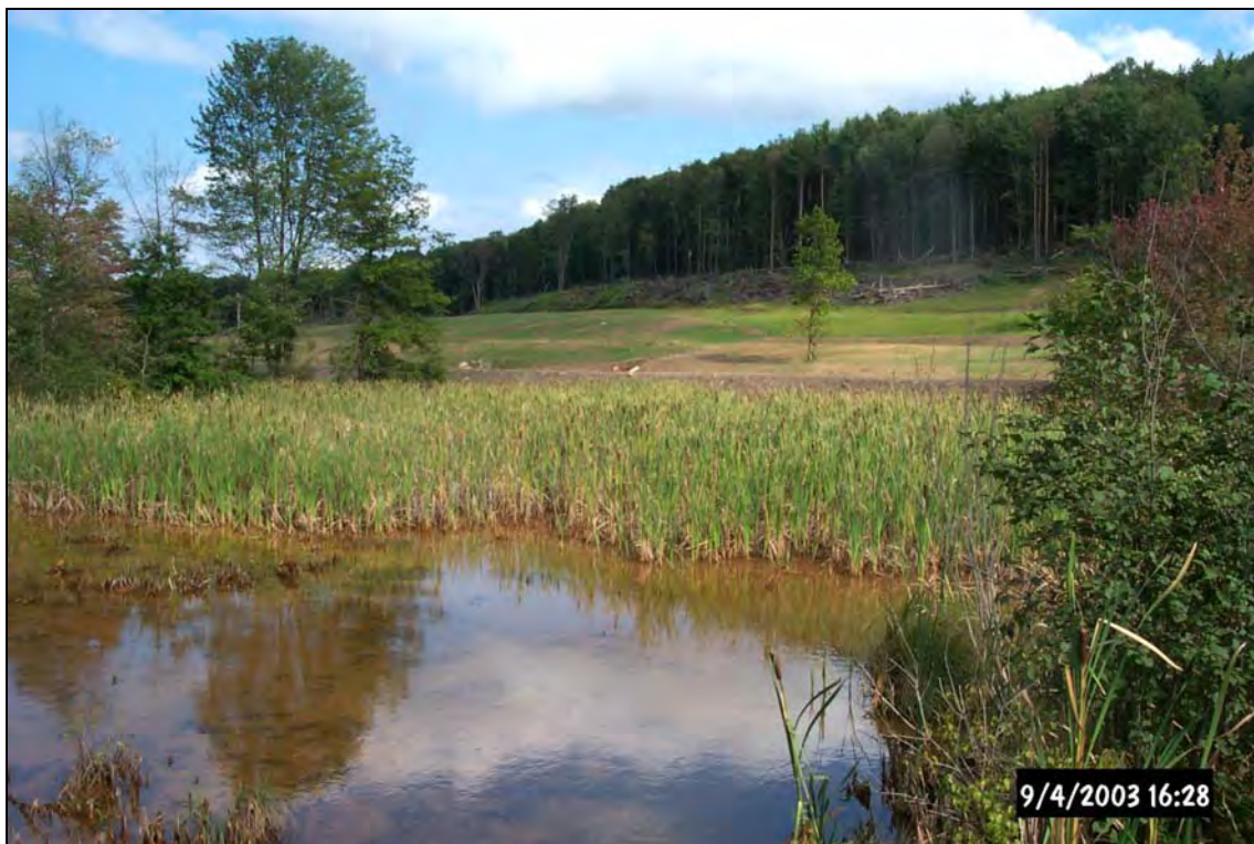
Anoxic Limestone Drain 3 (ALD3) discharges into Settling Pond 5 (SP5) (Above) which flows through the existing wetland before discharging into Seaton Creek (Below) .
