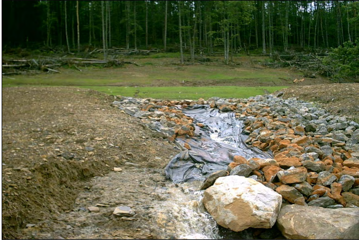
“Wash-out” (Above) on spillway from SP3 to WL2 resulted from severe storms. Following temporary repairs by Aquascape Intern Greg Holloway, Quality Aggregates, as part of in-kind contributions, repaired the spillway. Work and play (Below) on 7/29/03 during one of the many plantings with Butler County Juvenile Court Services: Working Opportunities to Repay the Community Program.
