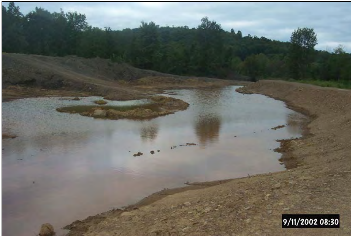
Views of the partially-excavated Wetland 2. Horizontal Flow Limestone Bed and ALD1 can be seen in the background of the photo below.
