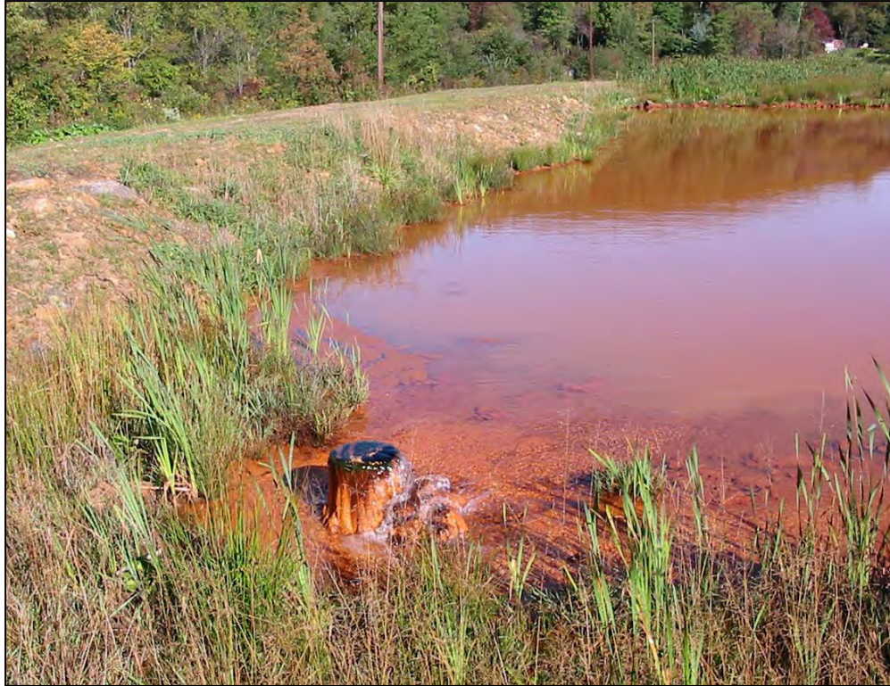
Anoxic Limestone Drain 2 (ALD2) discharges into Settling Pond 4 (SP4) (Above) which in turn discharges into Wetland 2 (WL2) via a rock-lined level spreader (Below) .
