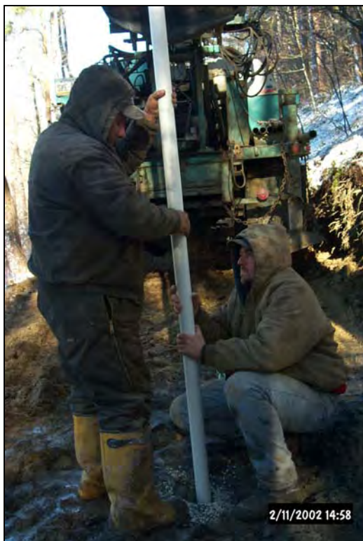
Mike and Jim from McKay & Gould Drilling Company worked with Margaret Dunn and Tim Danehy of BioMost, Inc. to install piezometers as part of the hydrogeologic investigation of the site for Passive Treatment System Design.
