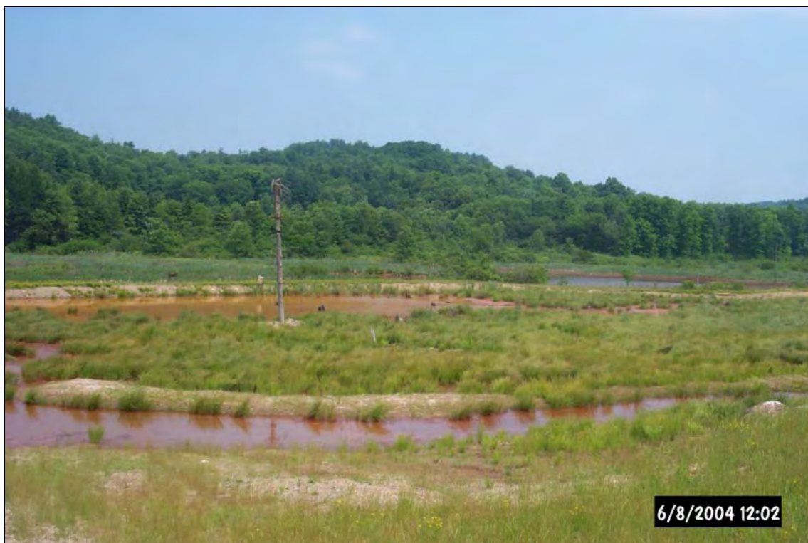
A seep zone ( Above ) located in the vicinity of pre-existing seeps flows into Wetland 2 near its outlet into the HFLB. A channel and berm ( Below ) were constructed to direct the water to the western end of WL2.
