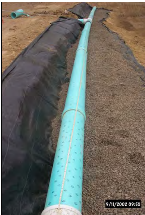
Anoxic Limestone Drain 1 (ALD1) included 8,300 tons of aggregate. The customized, effluent manifold piping system can be seen above and below.
