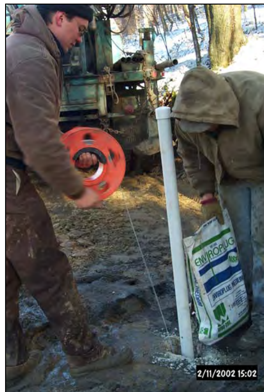
Mike and Jim from McKay & Gould Drilling Company worked with Margaret Dunn and Tim Danehy of BioMost, Inc. to install piezometers as part of the hydrogeologic investigation of the site for Passive Treatment System Design.
