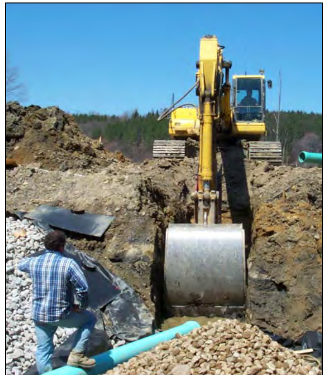
Construction of ALD2: Limestone aggregate has been placed. Non-reactive sandstone is being placed around ALD influent pipe and in several seeps to collect the discharge. Netting was placed around the pipe to prevent smaller-sized aggregates from entering perforations.
