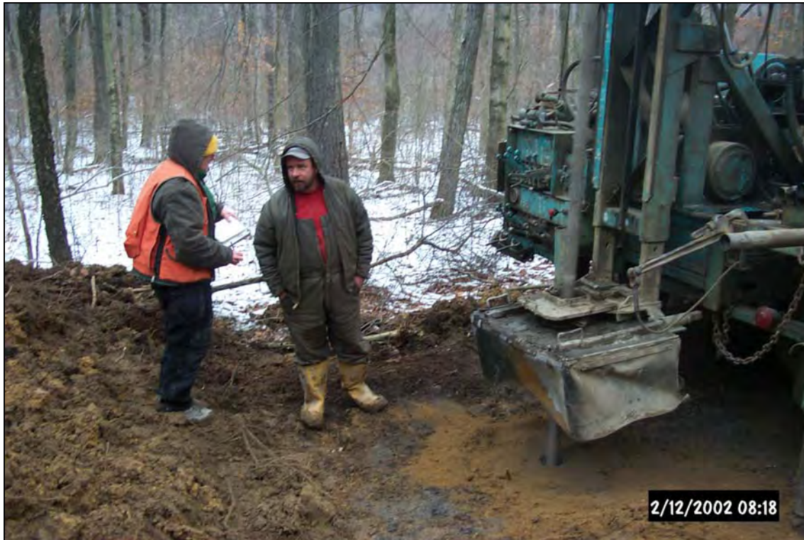
Mike and Jim from McKay & Gould Drilling Company worked with Margaret Dunn and Tim Danehy of BioMost, Inc. to install piezometers as part of the hydrogeologic investigation of the site for Passive Treatment System Design.
