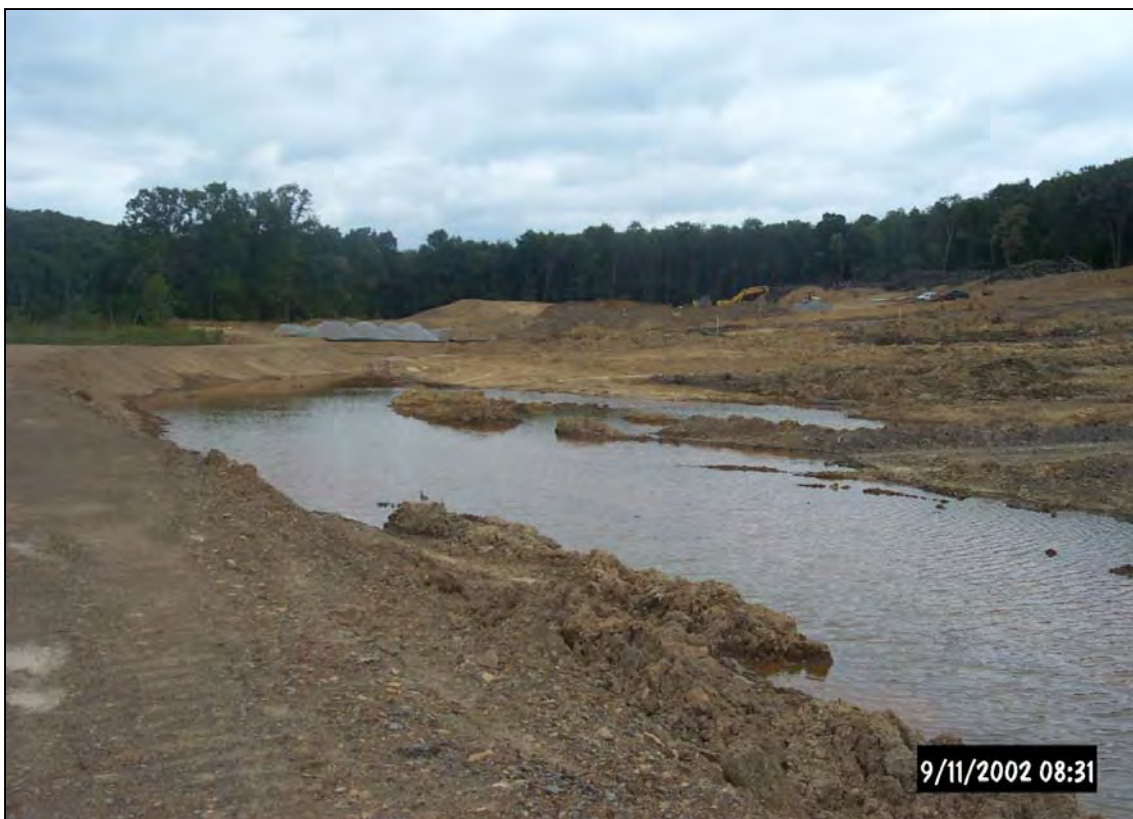
Views of the partially-excavated Wetland 2. Horizontal Flow Limestone Bed and ALD1 can be seen in the background of the photo below.
