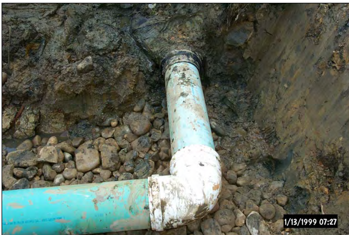
John Stoops and Wayne Fuchs ( Above ) of Quality Aggregates are cutting a section of pipe to be used in the ALD3 collection system. Piping was attached using a Fernco ( Below ) to the existing pipe that conveyed ST63A.
