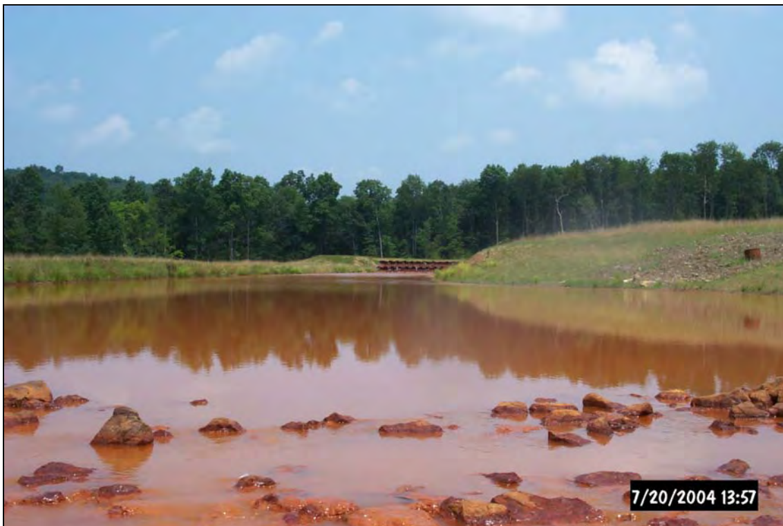
Settling Pond 1 (SP1) discharges into Settling Pond 2 (SP2) (Below) via the Z-piling and riprap spillway (Above) .
