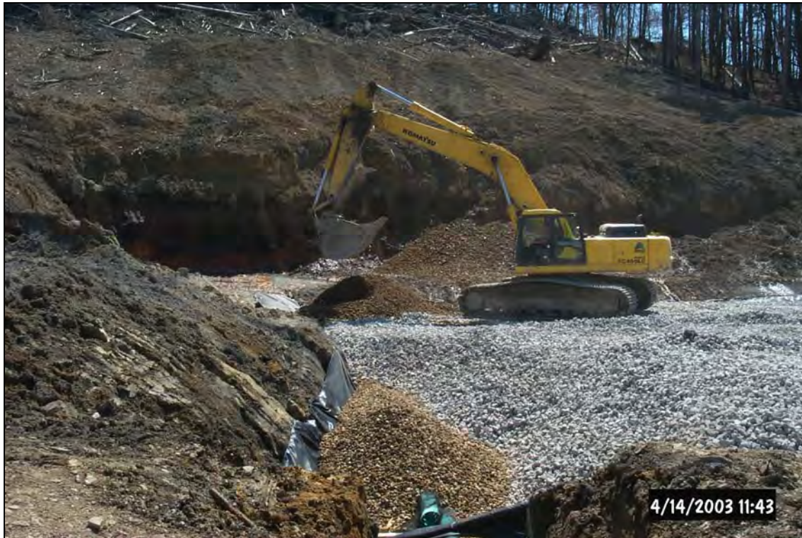
Construction of ALD2: Limestone aggregate has been placed. Non-reactive sandstone is being placed around ALD influent pipe and in several seeps to collect the discharge. Netting was placed around the pipe to prevent smaller-sized aggregates from entering perforations.
