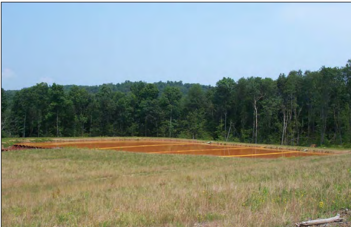
Anoxic Limestone Drain 1 (ALD1) discharges (Above) into Settling Pond 1 (SP1) (Below) . Three baffle curtains were installed to increase retention time within the pond in order to oxidize and hydrolyze as much dissolved iron as possible.
