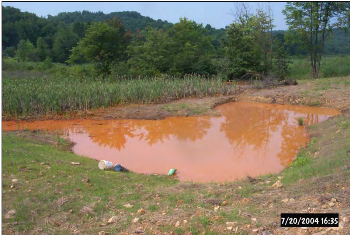
Anoxic Limestone Drain 3 (ALD3) discharges into Settling Pond 5 (SP5) (Above) which flows through the existing wetland before discharging into Seaton Creek (Below) .
