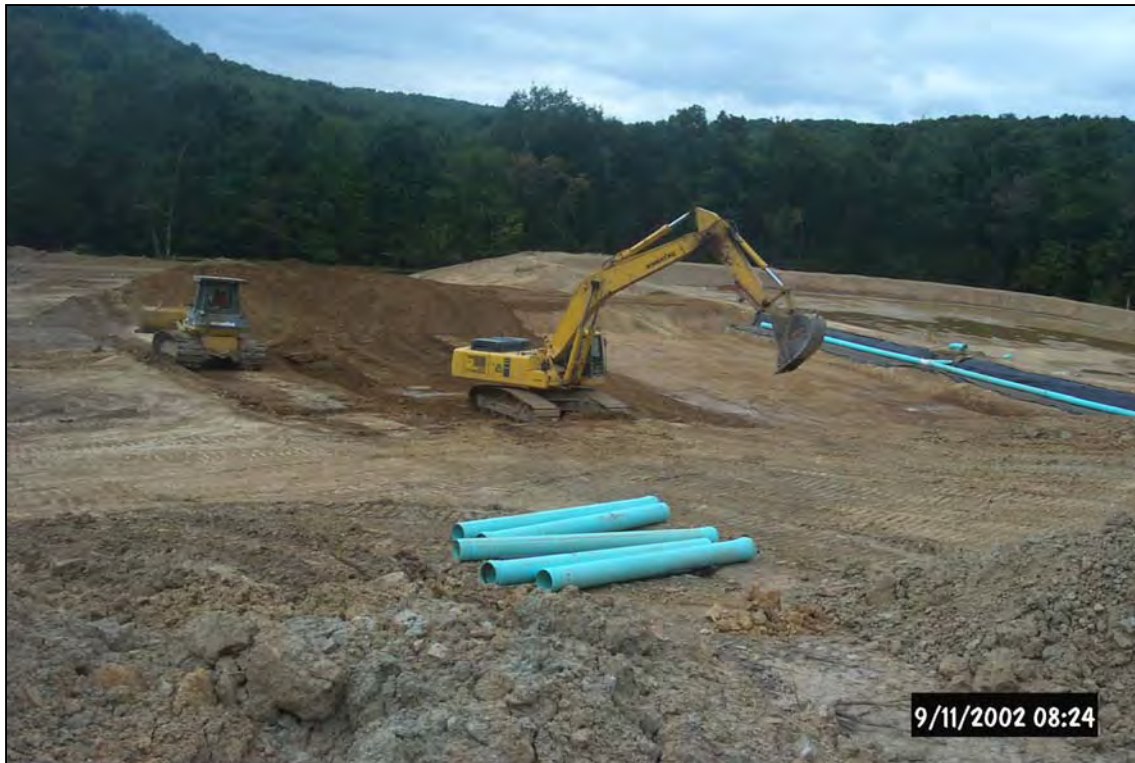
Anoxic Limestone Drain 1 (ALD1) included 8,300 tons of aggregate. The customized, effluent manifold piping system can be seen above and below.
