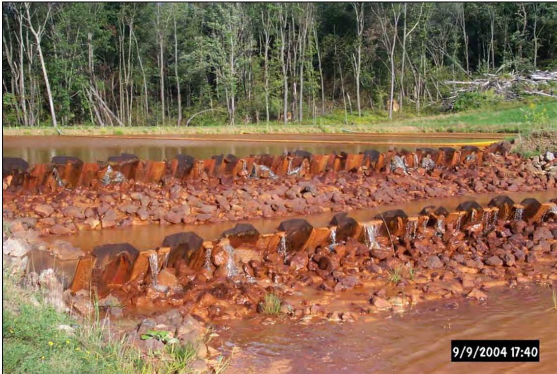
Settling Pond 1 (SP1) discharges into Settling Pond 2 (SP2) (Below) via the Z-piling and riprap spillway (Above) .
