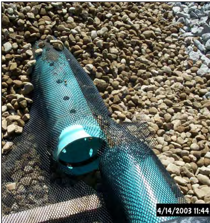
Construction of ALD2: Limestone aggregate has been placed. Non-reactive sandstone is being placed around ALD influent pipe and in several seeps to collect the discharge. Netting was placed around the pipe to prevent smaller-sized aggregates from entering perforations.
