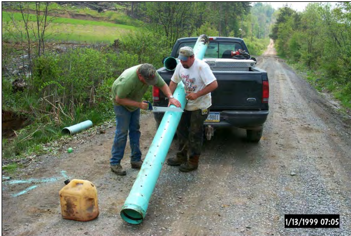
John Stoops and Wayne Fuchs ( Above ) of Quality Aggregates are cutting a section of pipe to be used in the ALD3 collection system. Piping was attached using a Fernco ( Below ) to the existing pipe that conveyed ST63A.
