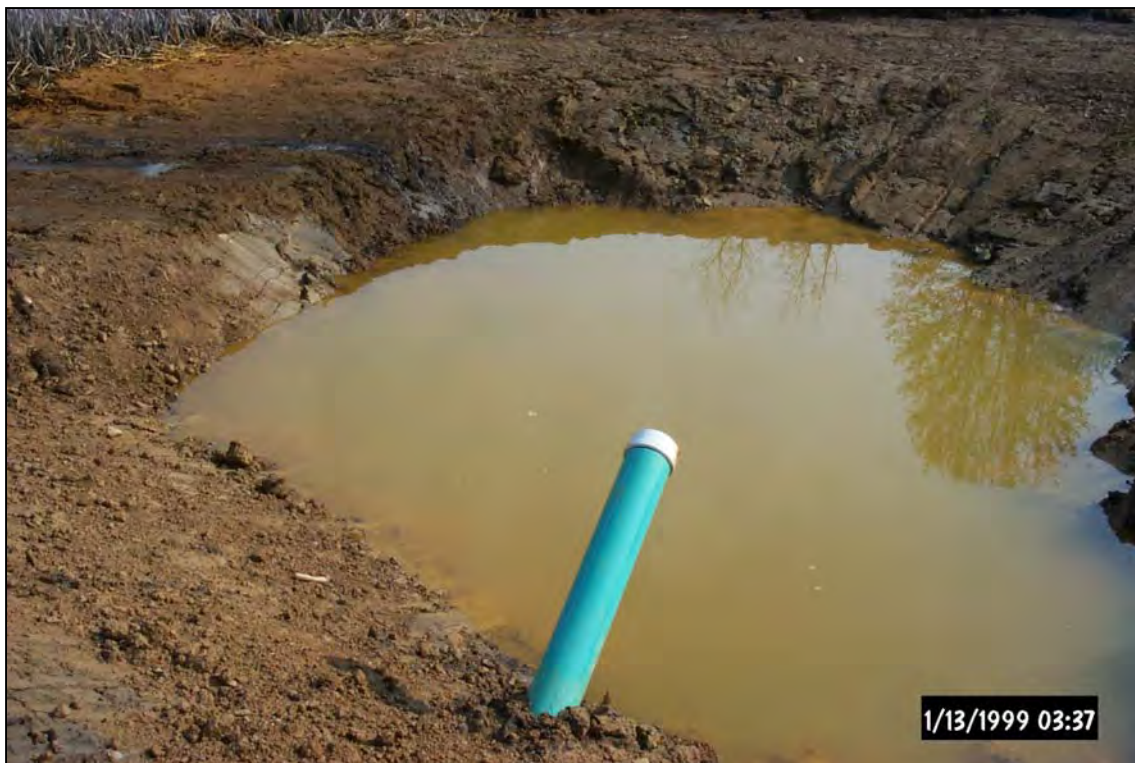
Above: 90% \text{CaCO}_3 , AASHTO#1, Vanport limestone placed within ALD3. Below: Effluent pipe capped until water turned into the system. Portion of Settling Pond 5 (SP5) completed.
