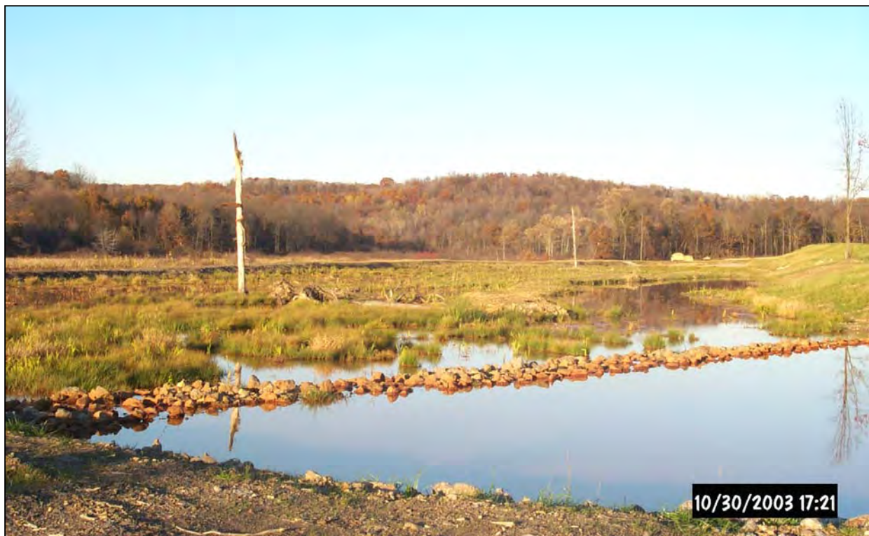
Anoxic Limestone Drain 2 (ALD2) discharges into Settling Pond 4 (SP4) (Above) which in turn discharges into Wetland 2 (WL2) via a rock-lined level spreader (Below) .
