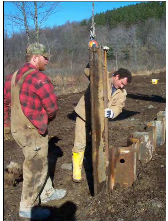
John Stoops, Mike Colosimo, and Kevin Stiner of Quality Aggregates installing Z-piling in order to maintain pre-project stream elevation from existing beaver dam across Seaton Creek at the “narrows” between the Flick and L-shaped gob piles. (3/28/02)
