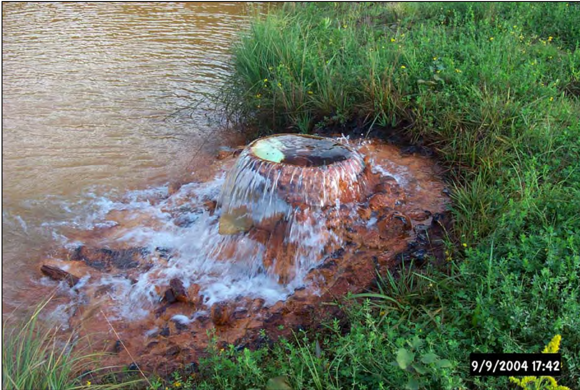
Anoxic Limestone Drain 1 (ALD1) discharges (Above) into Settling Pond 1 (SP1) (Below) . Three baffle curtains were installed to increase retention time within the pond in order to oxidize and hydrolyze as much dissolved iron as possible.
