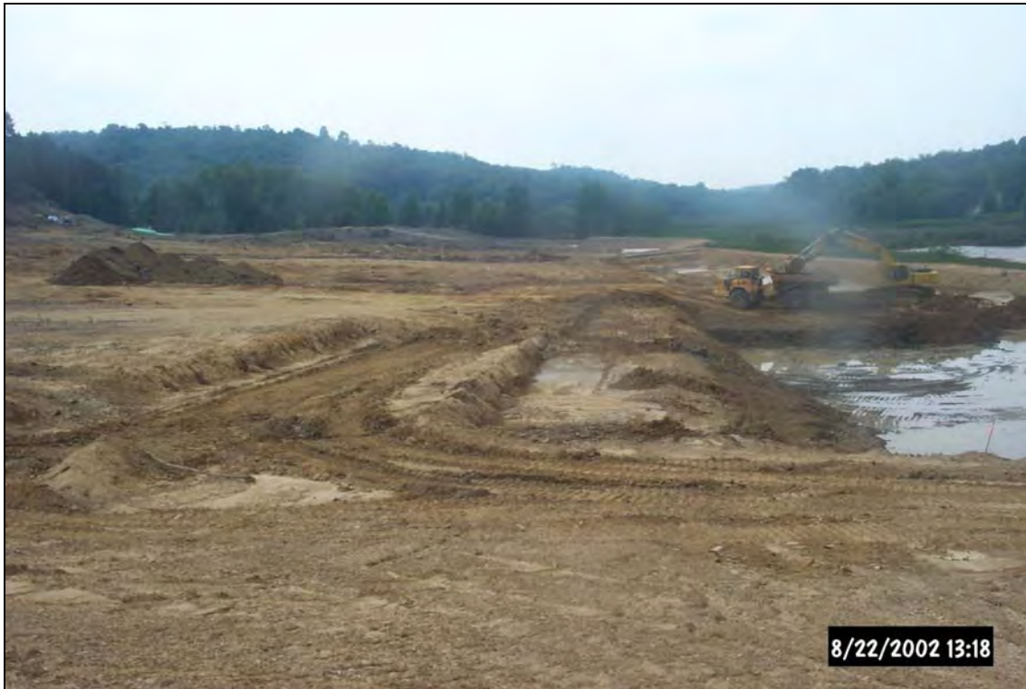
Excavation for Horizontal Flow Limestone Bed required substantial “dirt moving”.
