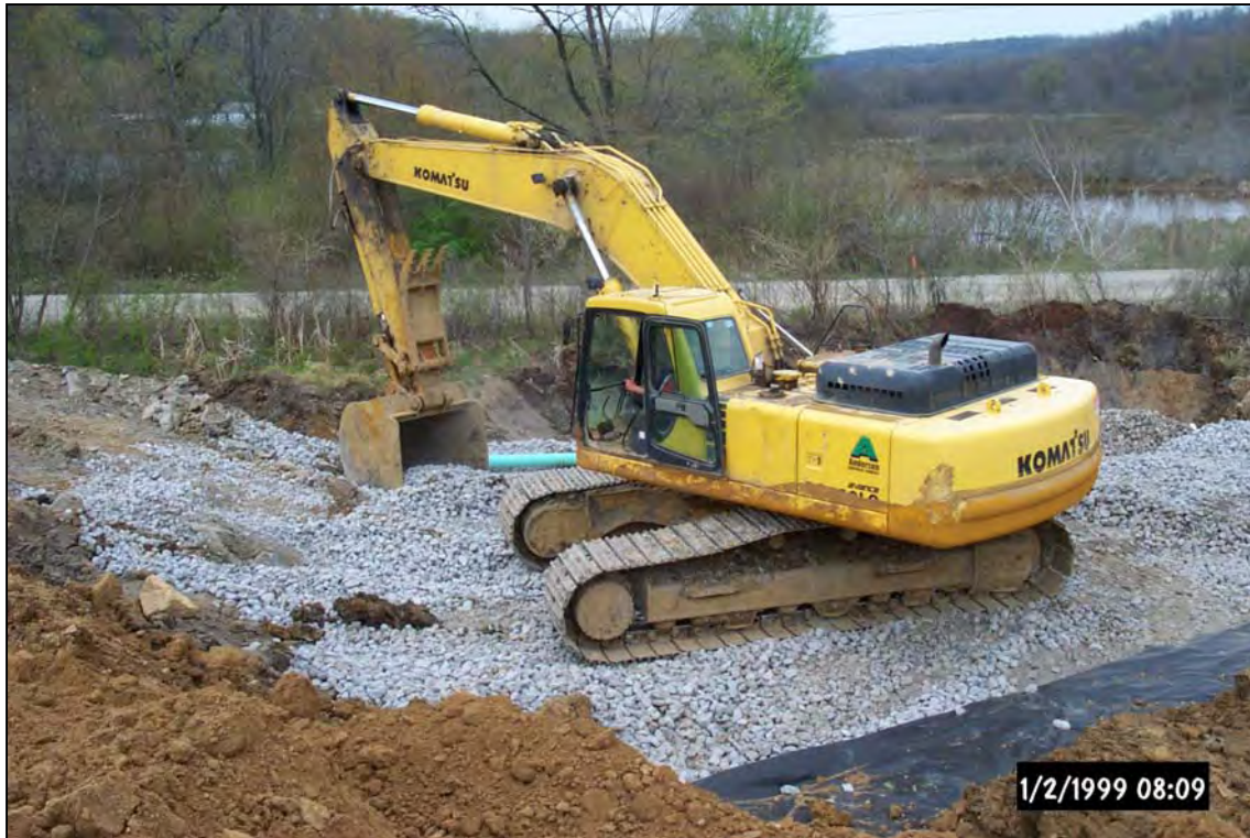
Above: 90% \text{CaCO}_3 , AASHTO#1, Vanport limestone placed within ALD3. Below: Effluent pipe capped until water turned into the system. Portion of Settling Pond 5 (SP5) completed.
