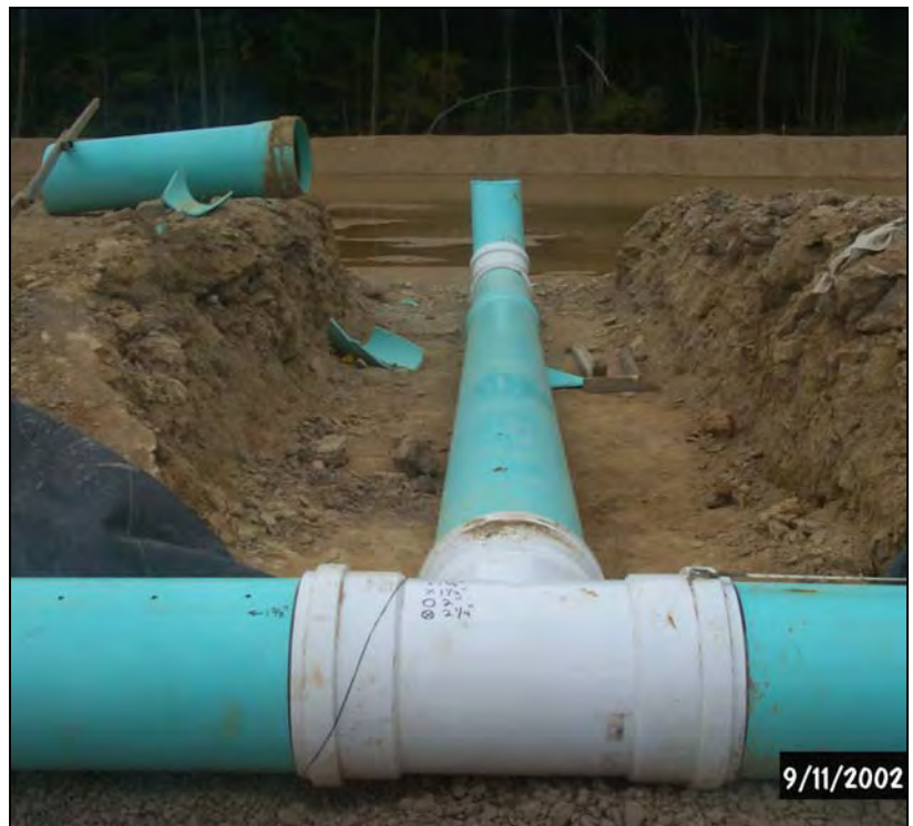
Anoxic Limestone Drain 1 (ALD1) included 8,300 tons of aggregate. The customized, effluent manifold piping system can be seen above and below.
