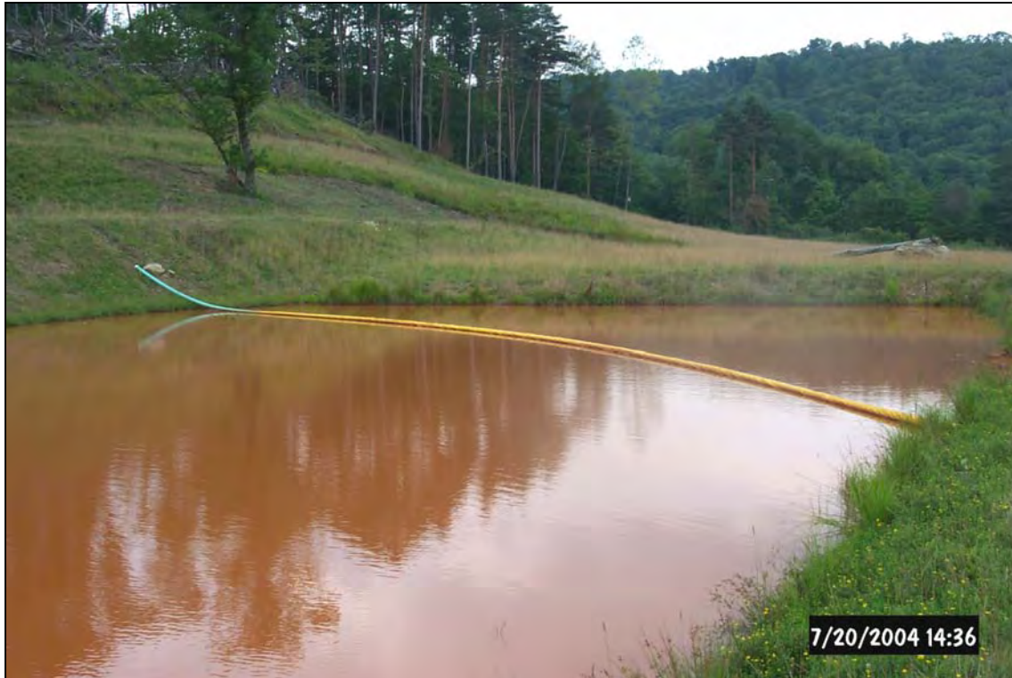
Settling Pond 3 ( Above ) receives influent from Wetland 1. A baffle curtain was installed to decrease short-circuiting and to increase retention time before discharging into Wetland 2 via a rock-lined spillway ( Below ).
