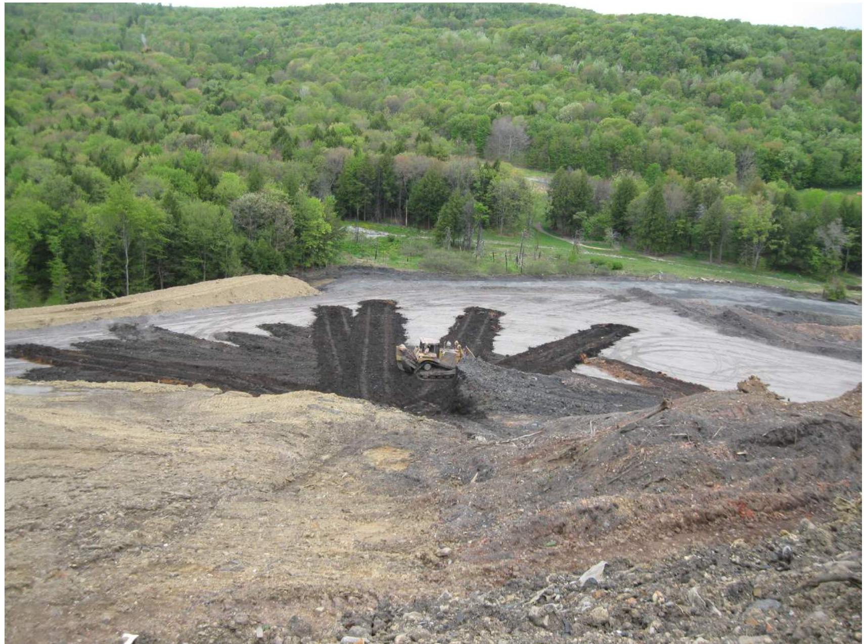
Reject refuse material being spread on top of a layer of ash Photo from Nanty Glo West on May 7, 2010
