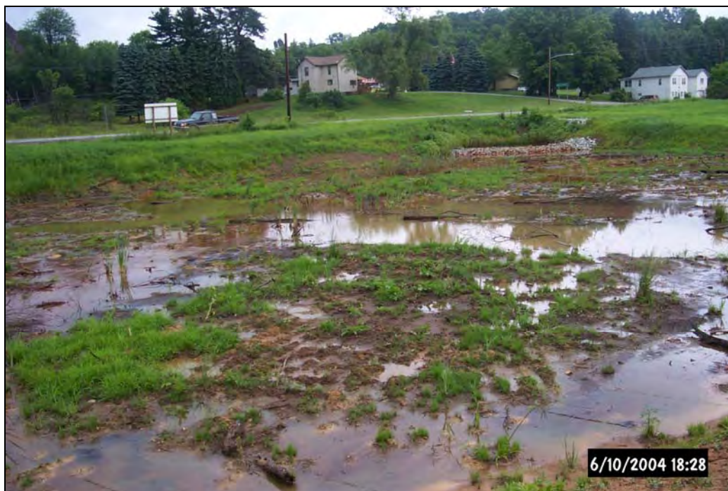
Wetland vegetation that was planted on 4/2/04 and has colonized naturally has begun to grow. The wetland was constructed with microrelief and several deeper pools to enhance the system performance for treatment and wildlife value.
