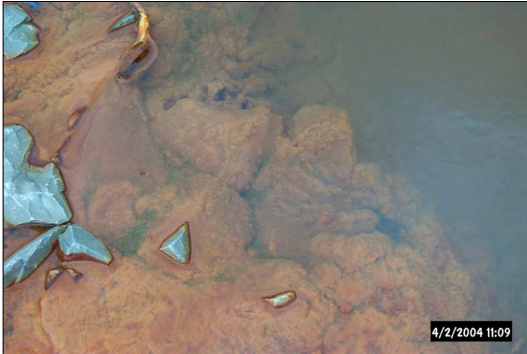
Iron has begun to thickly coat the rip-rap level spreader after only three months of operation.
