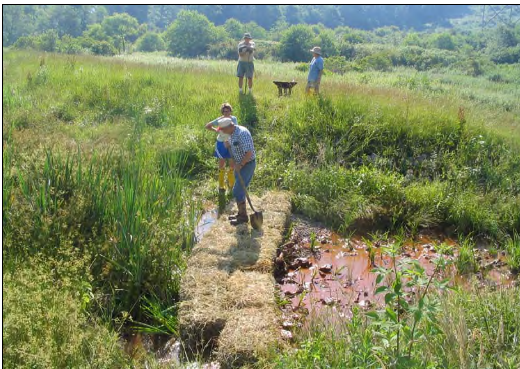
Hay bales were placed at the outlet of the wetland to encourage more uniform distribution of the mine discharge throughout the wetland.
