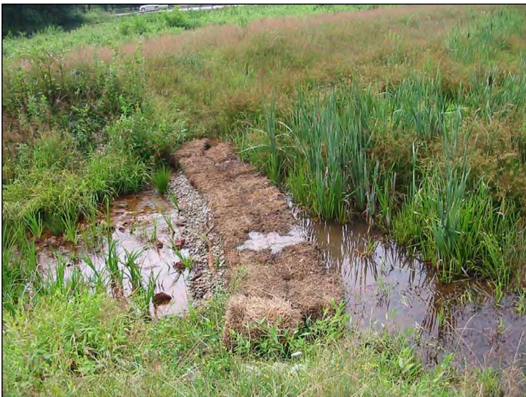
Rock was placed below the hay bales to help keep them in place. Notice that the water elevation is at the top of the of hay bales (below).
