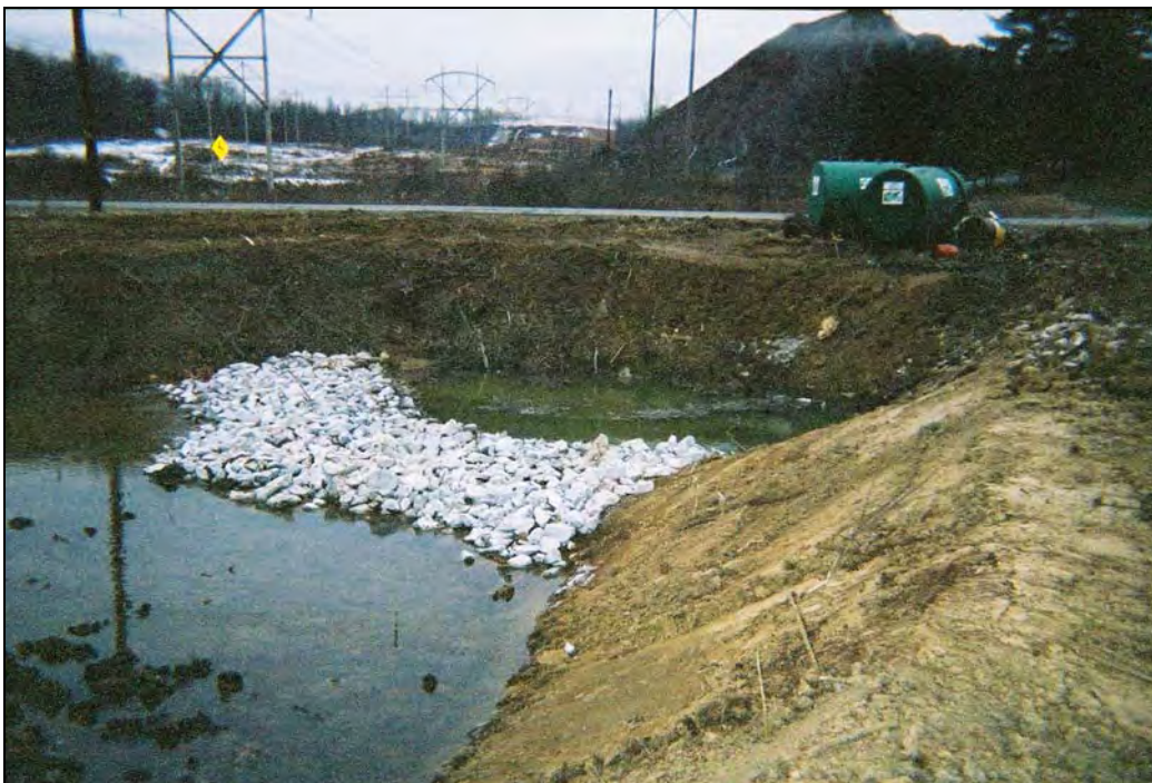
The forebay shortly after construction. The freshly laid limestone has not yet been coated with iron.
