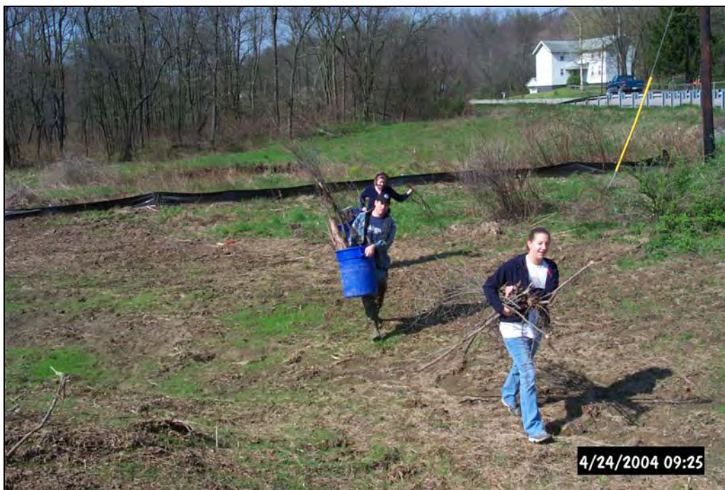
As part of the wetland planting, woody debris from the surrounding area was gathered and strategically placed throughout the wetland to add habitat diversity and help prevent preferential flow paths.
