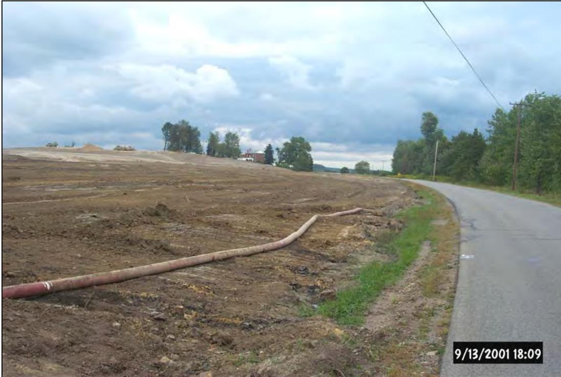
As part of the reclamation process, the acidic, abandoned mine drainage in the open pits was pumped to treatment ponds and chemically treated before discharging to an unnamed tributary to Wolf Creek.
