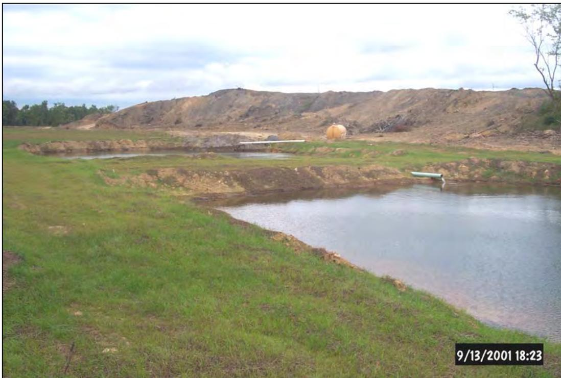
**Top:** View of the temporary treatment ponds used while pumping acidic, abandoned mine drainage from open water-filled pits.
