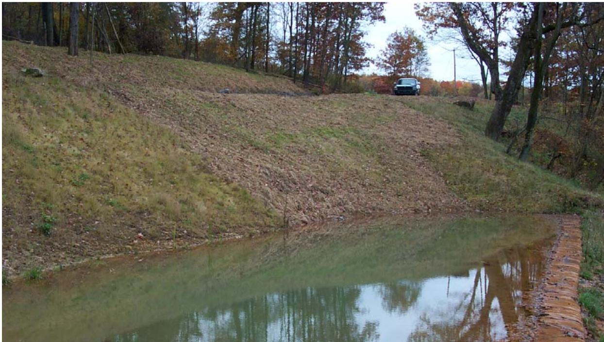
OSM Funding was used to install a French drain upgradient of the cut slope to intercept the subsurface flow, install buried limestone riprap reinforcement and successfully stabilize the slope. (10/20/04)
