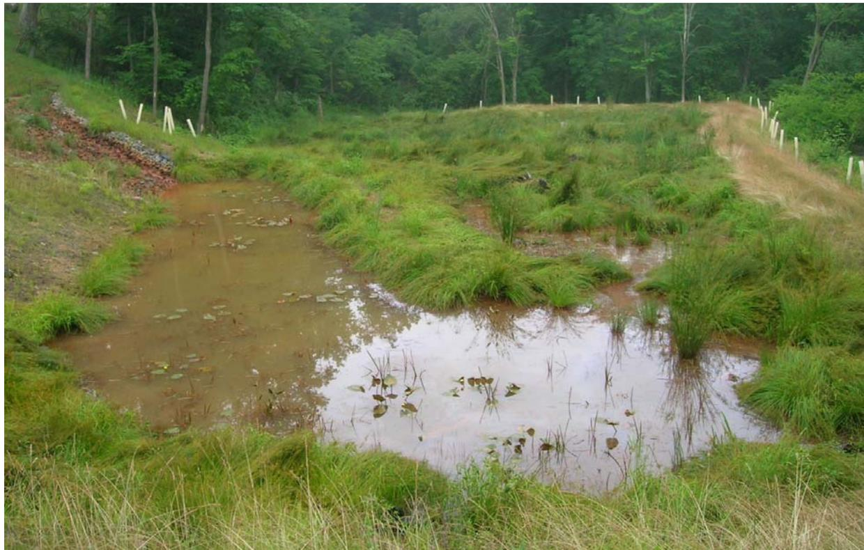
Settling pond (to left of photograph) outlets via an aeration spillway (top left) into a drop pond area (left and foreground), flows into the aerobic wetland and outlets to Semiconon Run near the top center of the photograph. System currently reduces iron concentrations from 22 mg/l to less than 3 mg/l.
