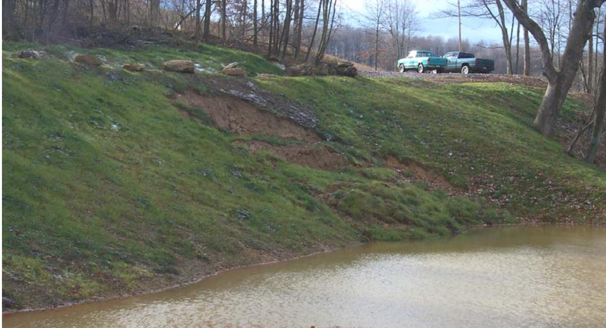
Slumping occurred above the settling pond due to significant shallow subsurface flows that were likely exasperated by heavy precipitation. (11/13/03)
