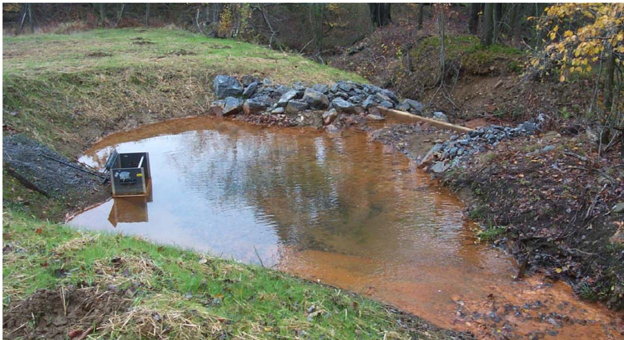
OSM funding was used to install a stream intake-type collection system that directs the abandoned mine drainage into the passive system. (10/20/04)
