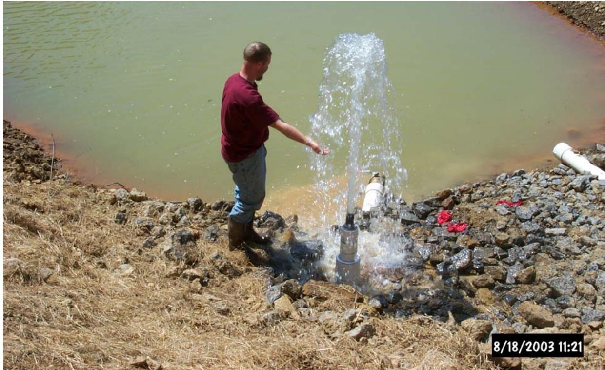
After the initial buried collection systems were installed, the discharge was successfully collected and directed into the passive system. Vigorous agitation and aeration was achieved using the available hydraulic gradient. The system functioned very well through the fall of 2003.
