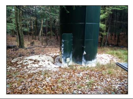
The Bear Run Phase 6 lime doser had become plugged with hardened lime caused by a previous flooding event. An attempt to clear the blockage with a power snake was ineffective. The lime had to be removed by hand through a removal observation panel.
