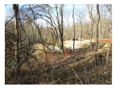
The DLB system is not quite complete. The concrete work is done but the 450 tons of limestone aggregate has not been delivered due to the weather. The bed is 4.5 ft deep and approximately 20 ft. by 100 ft. The sizing is based on the highly conservative assumption of 15 gpm flow and acidity removal. This conservative design was utilized so that its effectiveness will be assured and so that cleaning of the limestone should only be necessary every 10 years.
